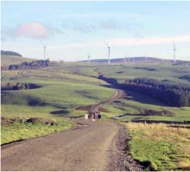
Garreg Lwyd wind farm under construction
