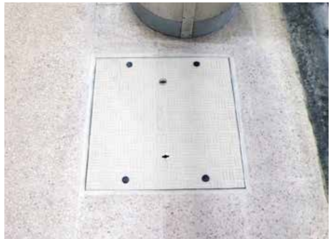
Fibrelite's bolted covers prevent unauthorised access
