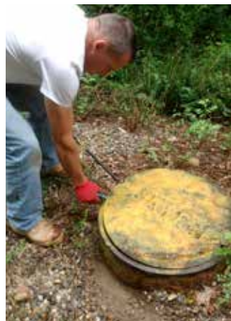
Heavy cast iron covers pose a significant threat of back & shoulder injuries along with the risk of trapped extremities
