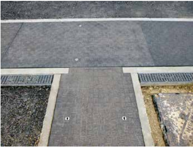
Fibrelite trench covers were retrofitted into existing precast concrete trenches
