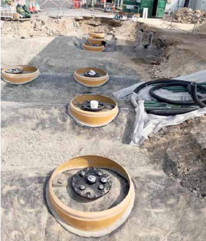
Fibrelite collars bonded ready for chamber installation
