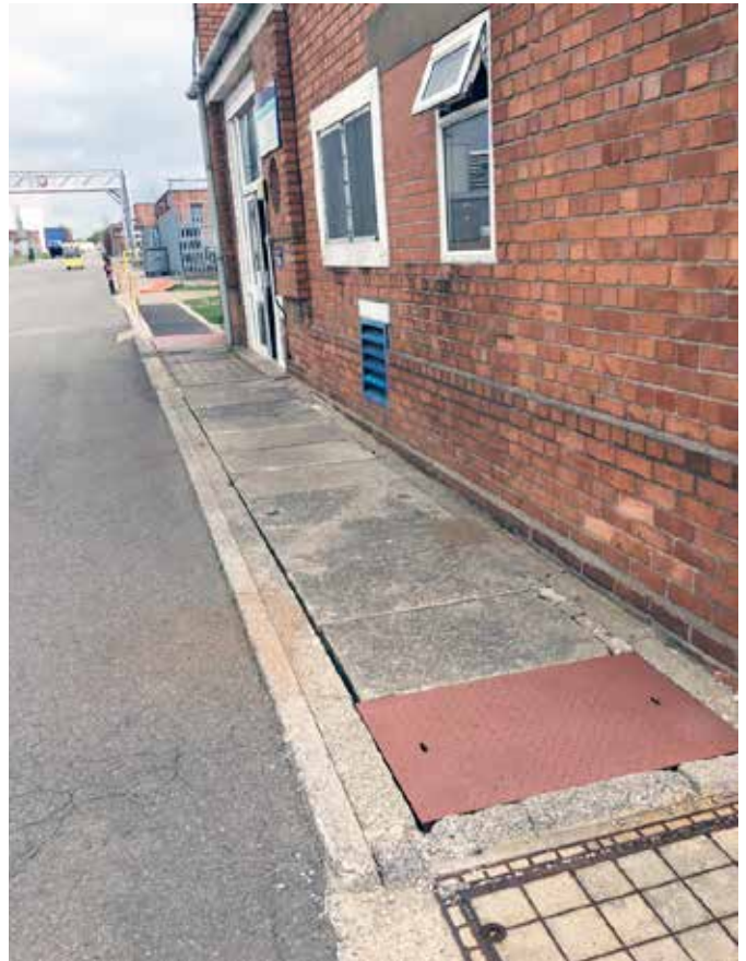
Previously installed covers had cracked and corroded
