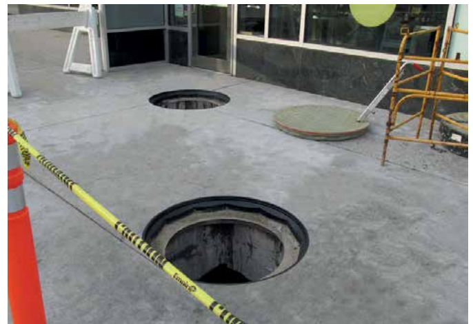
Fibrelite F95 composite cover installed in frame
