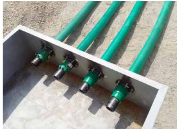
Training enabled a confident quality installation
