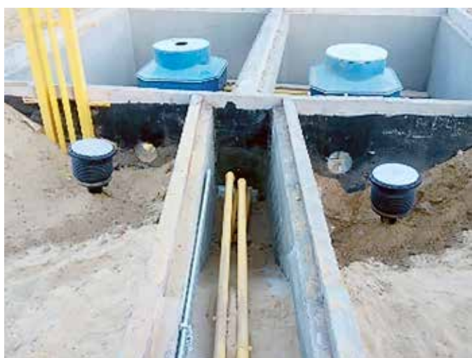
Fibrelite chambers and manhole covers provided an easy-install solution
