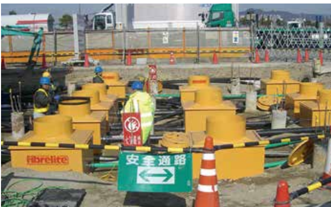
Vacuum tested tank sumps
