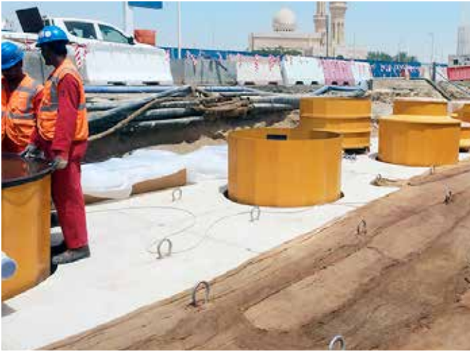
Fibrelite tank sump being vacuum tested on site
