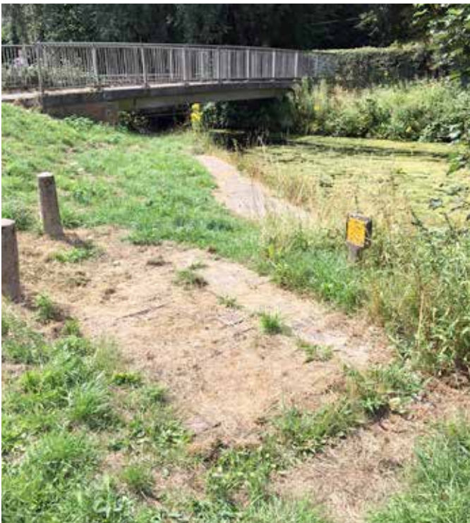
Previously installed covers had begun to degrade/rust
