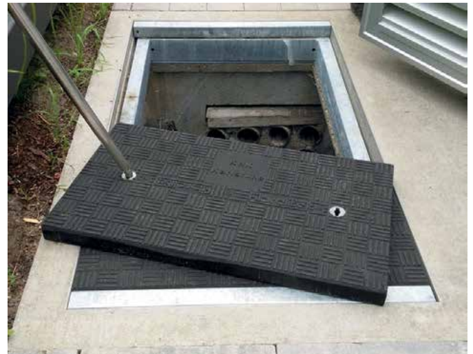
Fibrelite trench panels installed over the chamber
