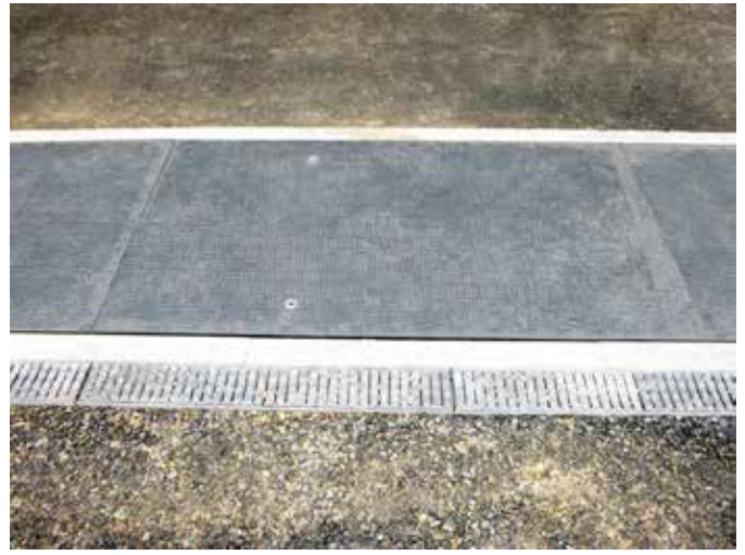
Vehicles operating onsite can now traverse the covers
