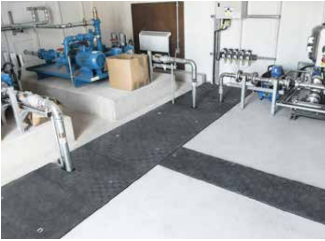
Two different load rated covers were used for the installations, B125 and D400
