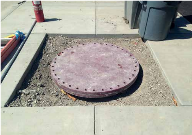
Fire protection tanks
