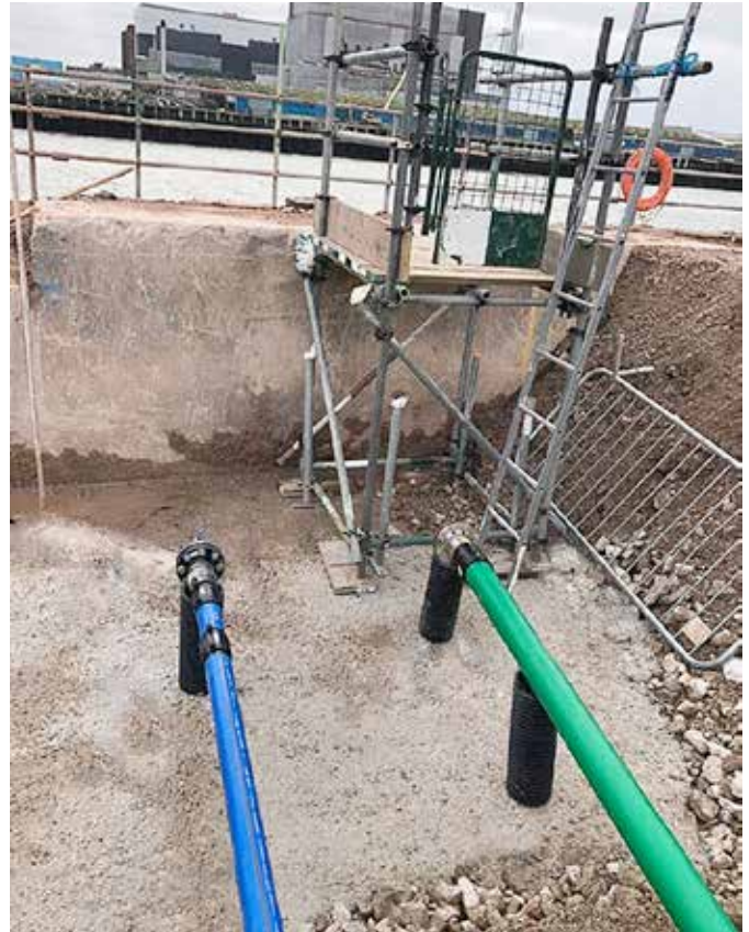
In house and onsite training was provided by OPW
