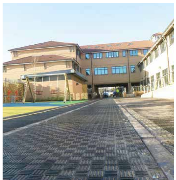
Fibrelite covers were manufactured at load ratings appropriate to their location
