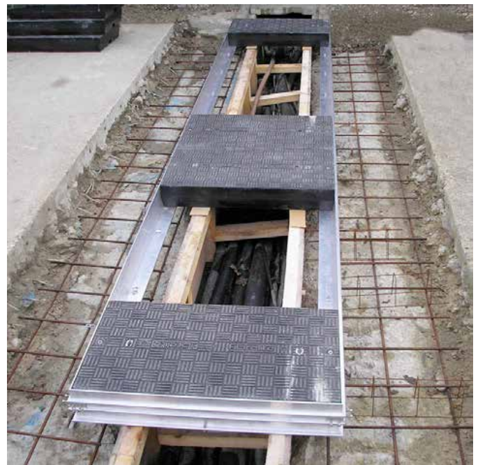
Fibrelite composite trench covers and aluminium frame during installation
