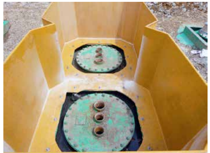
The new custom chambers provide a liquid-tight solution
