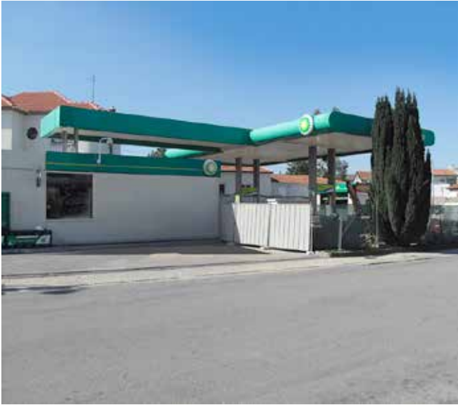
Site being upgraded with Fibrelite's fully conductive below ground remote fill sumps, covers and KPS conductive double wall fill pipe
