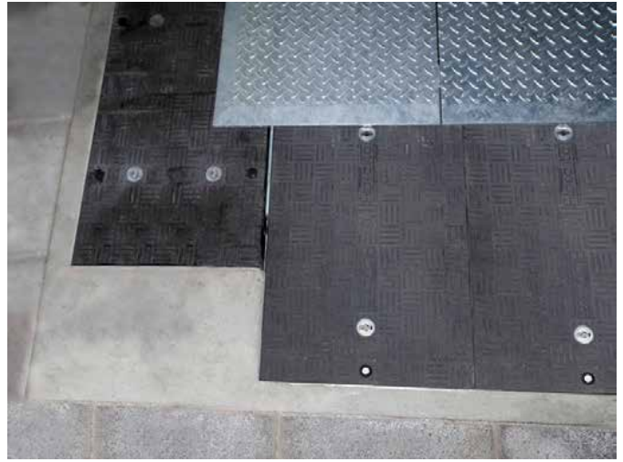
Securing system moulded into covers which locks into frame, preventing unauthorised access
