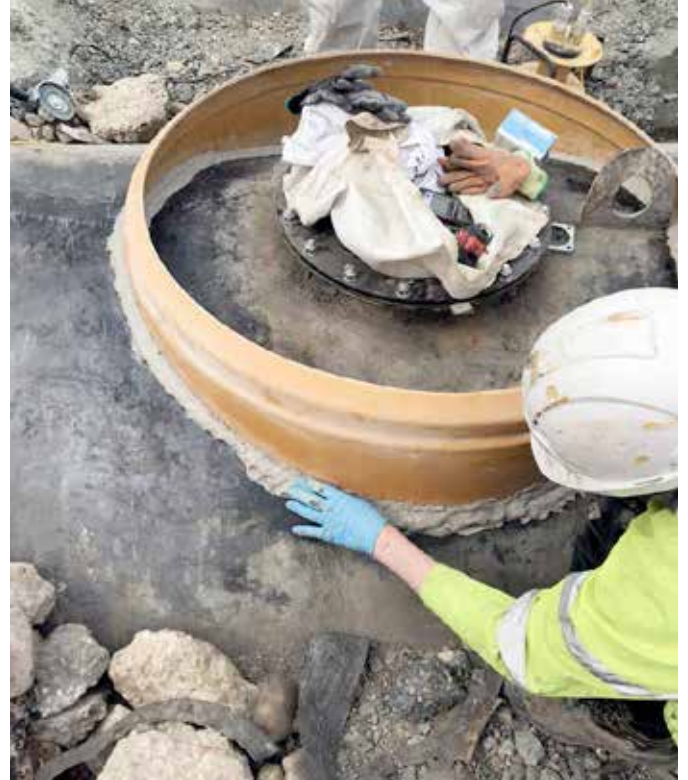
Bonding of the collar to the tank
