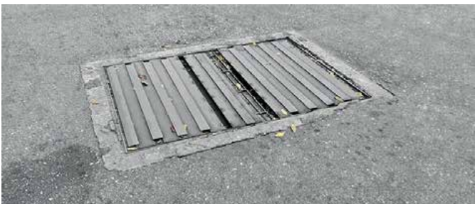
Previously installed steel access pit over water mains valve
