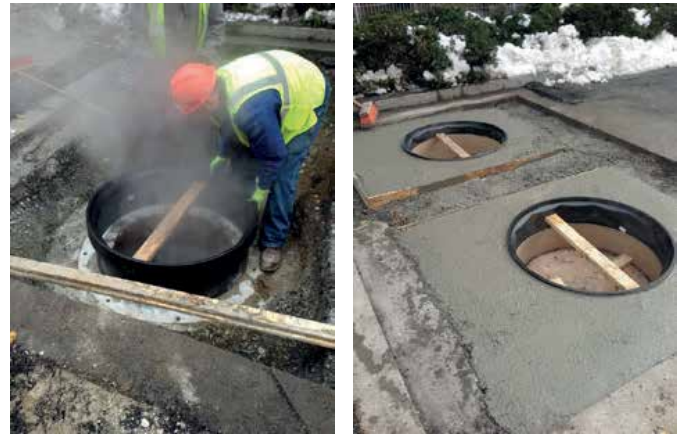
Fibrelite installations are simple – a fiberglass skirt can be used as a preform and to set the frame at grade
