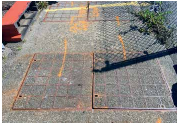
Covers were very heavy, making them time consuming to remove
