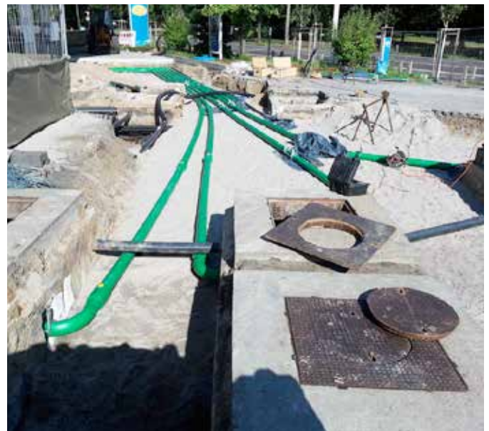
A key requirement of this project was limited downtime
