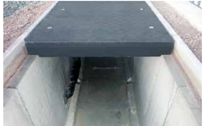
Covers 'stepped' to reduce weight and fit trench width
