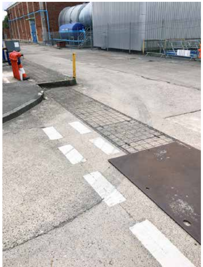
Covers were extremely heavy, requiring specialist equipment to remove
