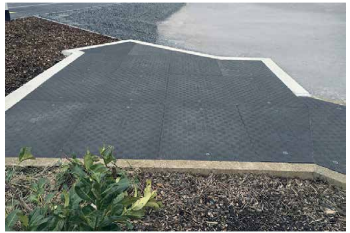
Covers supplied moulded to shape in the Fibrelite factory and supplied as a complete unit ready for installation
