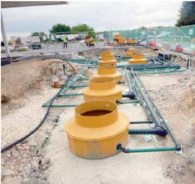
Fibrelite chambers bonded directly to previously installed fuel tanks upstands
