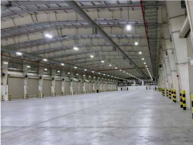
Fibrelite trench covers were specified for a support site in Bahrain
