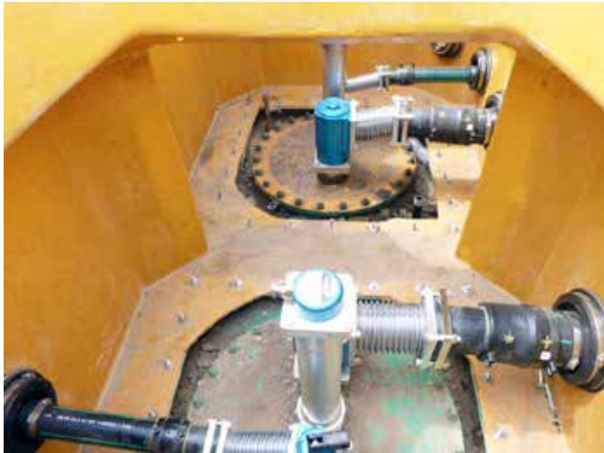
Fibrelite chambers were vacuum tested post-installation
