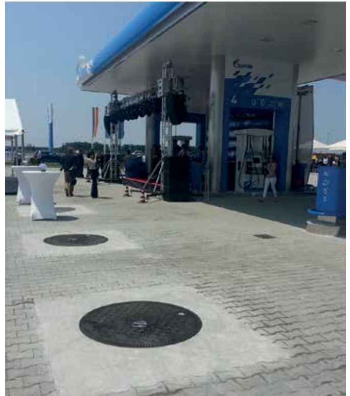
Fibrelite's FL100/CD cover. The central dip cover makes it easy to access the riser without having to remove the whole cover
