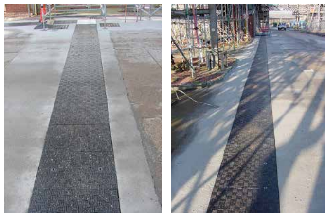
The senior designer on site commented that everyone was very pleased with the finished result
