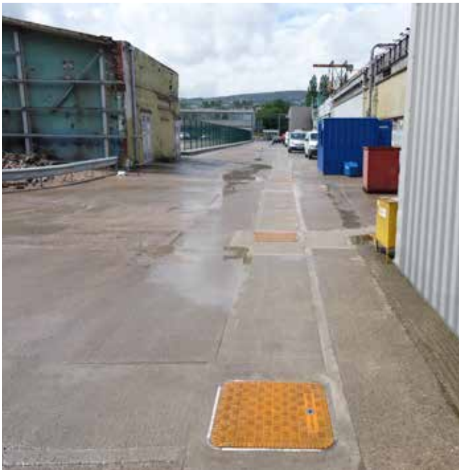
Heavy duty Fibrelite FL60/D400's
