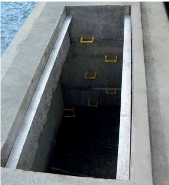
Access pit along edge of quay
