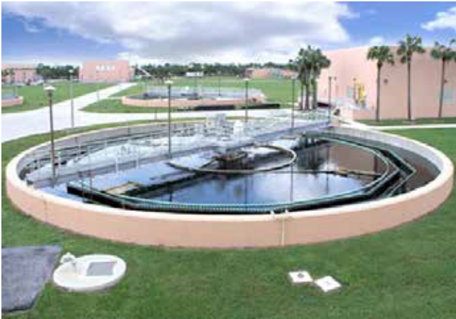
Concrete to Composites
