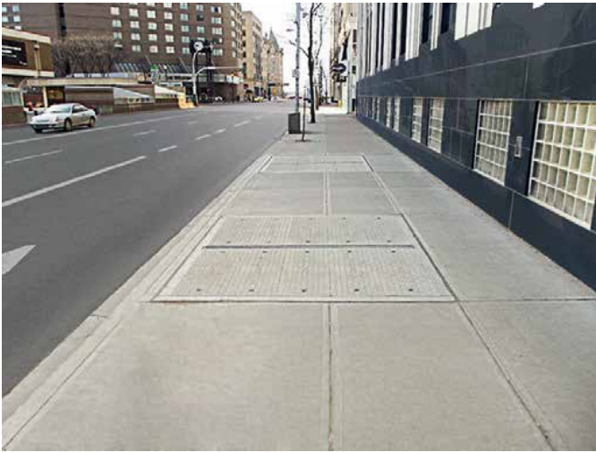
Finished cover installation in Edmonton
