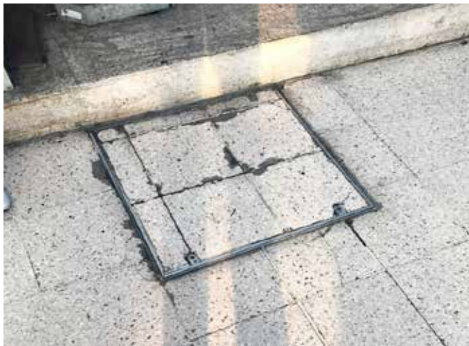
Colt construction were carrying out a platform upgrade programme
