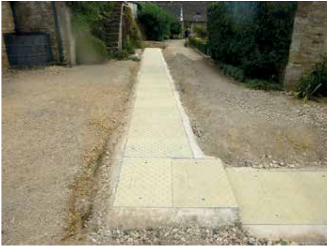
Fibrelite engineered and manufactured bespoke GRP trench covers for this countryside manor
