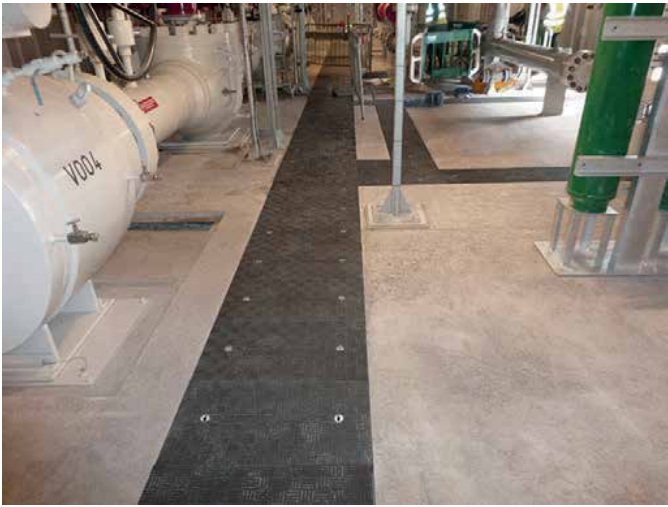
Non slip coating is applied to the top of the panels
