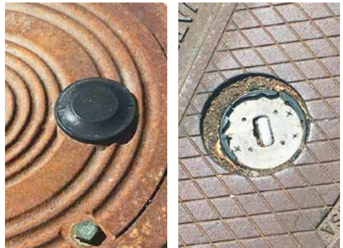
Previously installed metal covers exposed the antenna above the cover in order for the system to work
