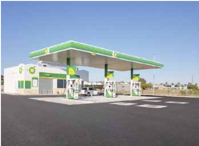
A suite of Fibrelite and KPS products eliminated potential installation issues and streamlined site construction at this Spanish site
