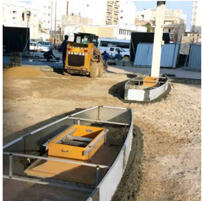
Fibrelite EL-G-E500 dispenser sumps ready for concreting
