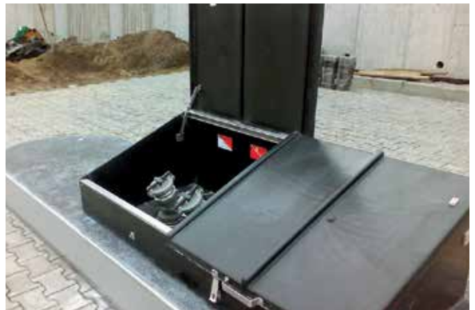
Vacuum testable GRP sump prevents water ingress from above or below ground
