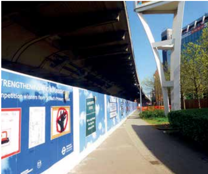
London Hammersmith flyover during refurbishment
