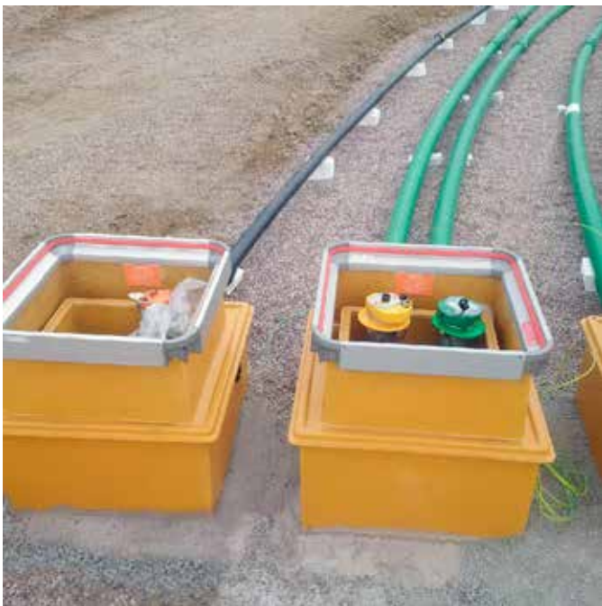
New sump and corbel utilised some items from existing product range to deliver a unique while cost effective solution
