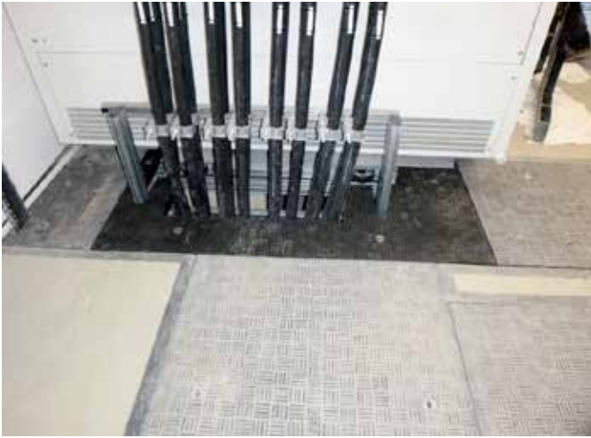
Fibrelite's GRP composite trench access covers can be easily and safely manually removed by two people
