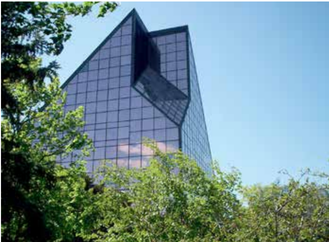
Fibrelite covers enable safe easy access to under floor utilities at the Royal Canadian Mint
