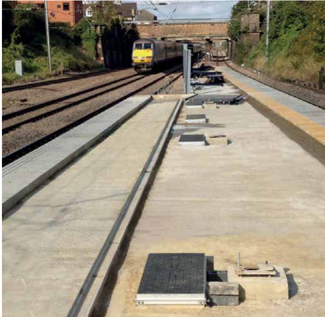
Section of train station platform with 4 covers (mid-way through install)
