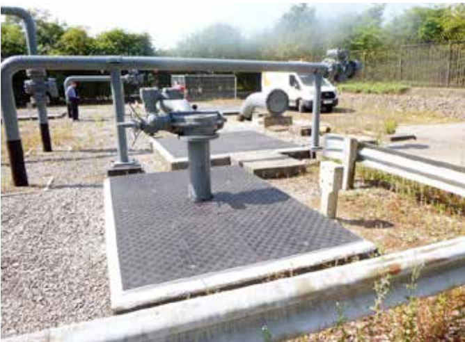
Covers were custom cut to accommodate existing valve network
