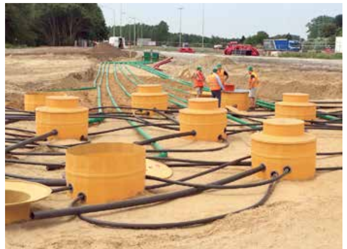
Fibrelite sumps and KPS piping reduced installation time
