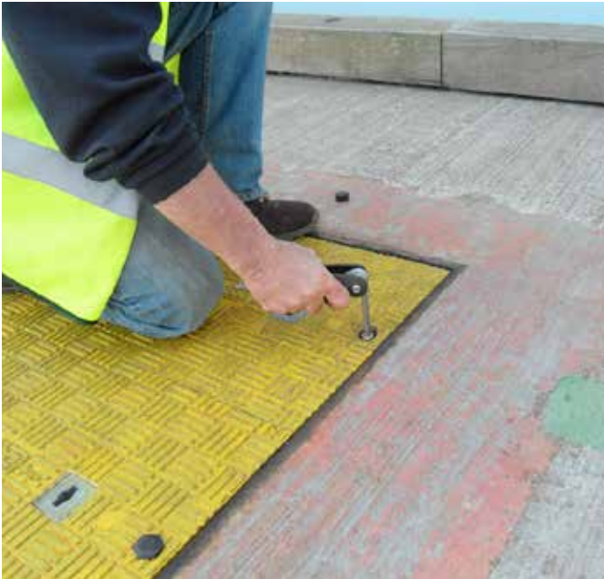
Operator removing the Fibrelite securing system
