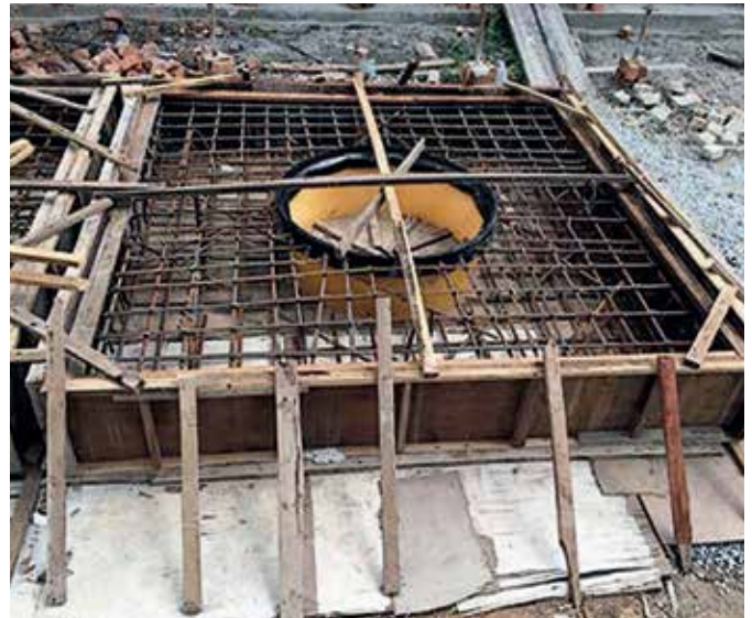
Prefabricating concrete plinth with Fibrelite FL90 frame
