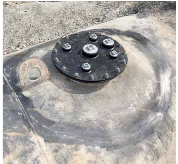
Preparation of the steel tanks and collar was key
