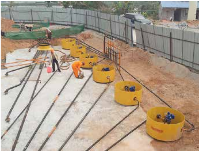
Fibrelite tank sumps (S14-390) being installed
