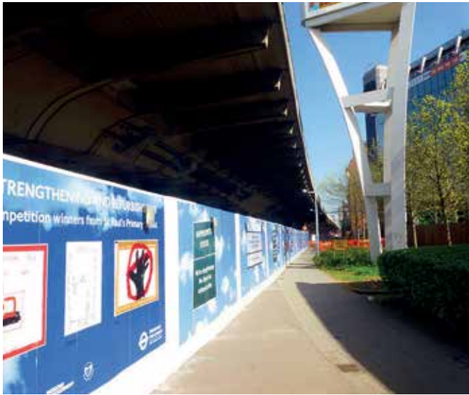
London Hammersmith flyover during refurbishment
