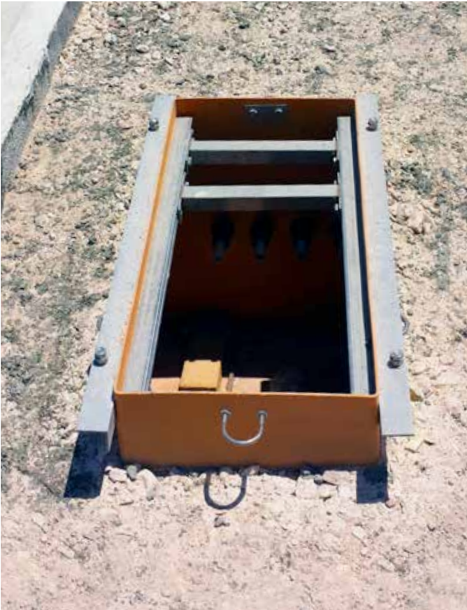
All Fibrelite sumps are vacuum testable during and after installation
