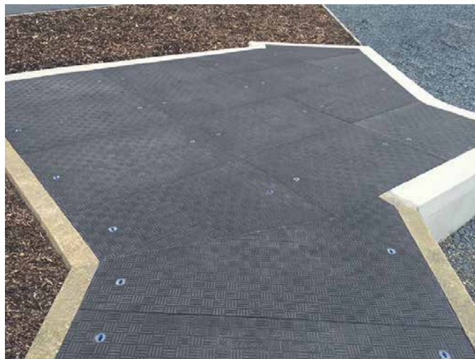
"Cassette" of bespoke covers over culvert
