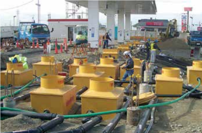
Fibrelite tank sumps and dispenser sumps being installed
