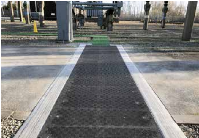
D400 load rated covers can be safely removed by two people
