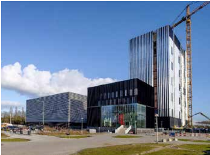
Fibrelite trench covers protect fibre optic cabling at emergency vehicle access point (image used for illustration purposes as actual data centre cannot be shown)
