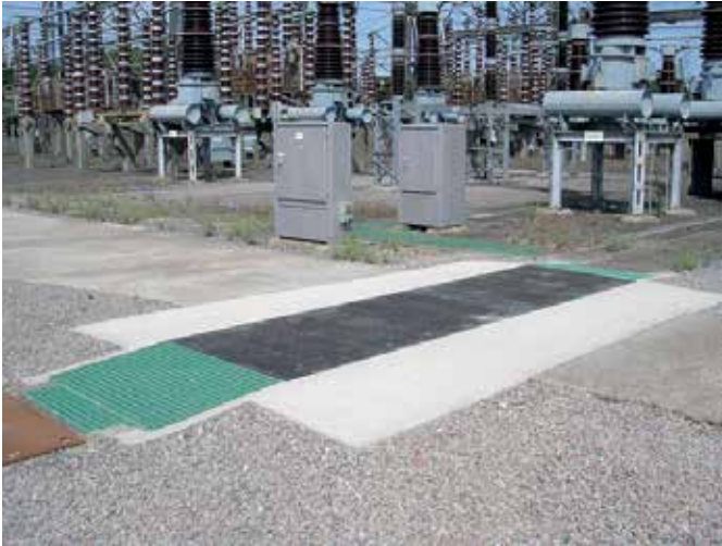
Fibrelite D400 tonne load rated lightweight trench covers
