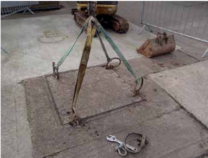
Lifting equipment required to remove heavy concrete covers
