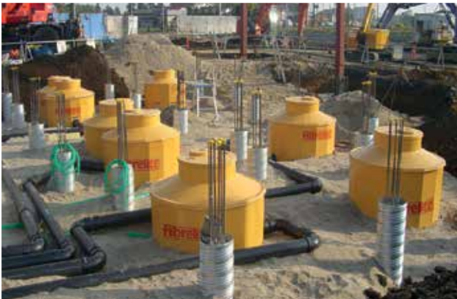
Fibrelite's 1.4m 16 sided tank sumps being installed
