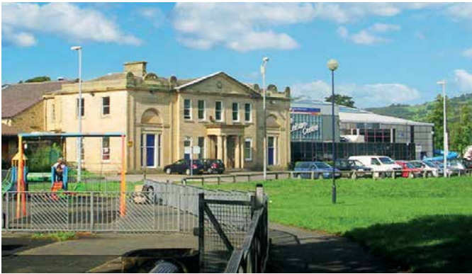
Fibrelite cover chosen for poolside at local leisure centre (Image credit: Betty Longbottom)
