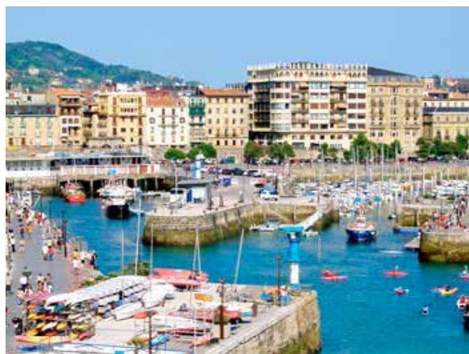
Ports Ondarreta, Sada and Malpica required KPS piping
