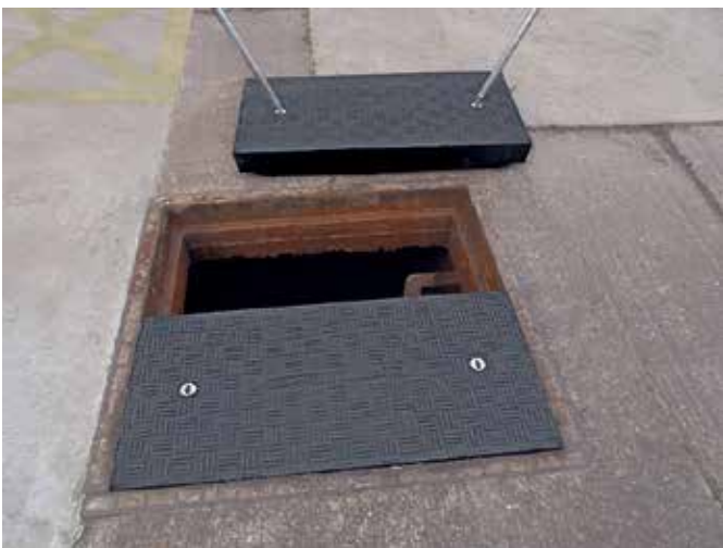
Bespoke Fibrelite covers installed into existing frame
