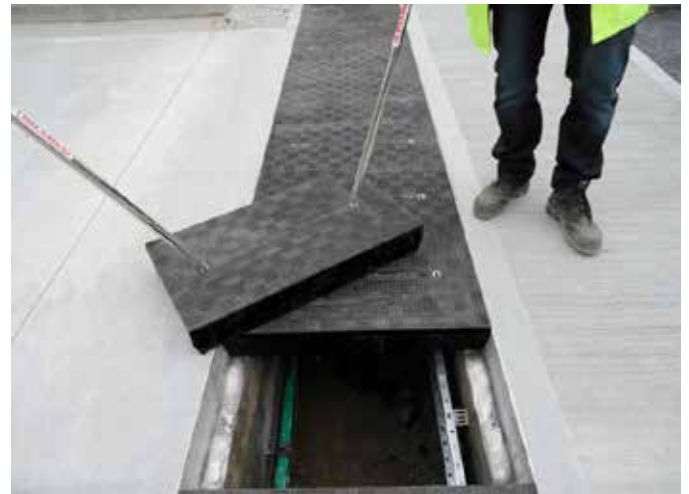
Fibrelite covers are designed to withstand heavy loads and harsh weather conditions for many years (Image of a similar installation used for illustration purposes as actual data centre cannot be shown)
