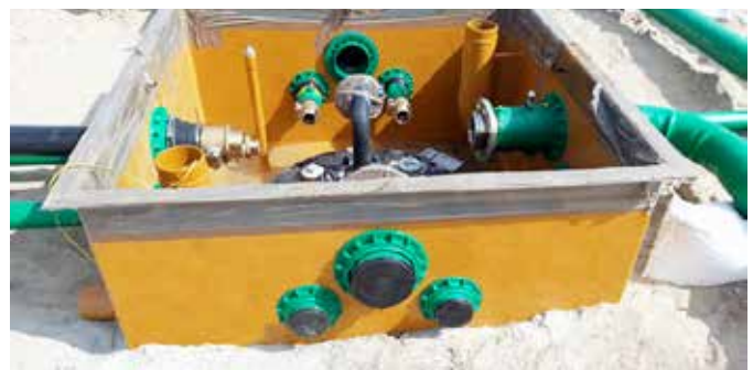
Tank chambers were supplied with pre-made holes on all chamber walls
