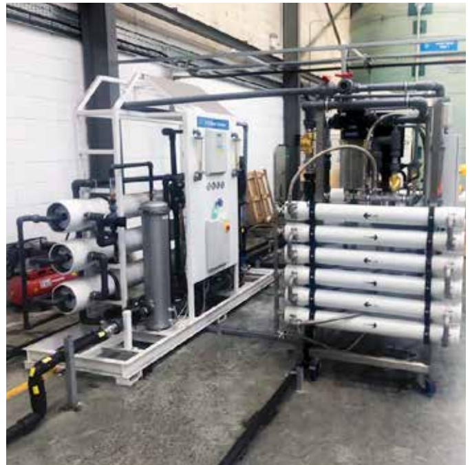
The installation was completed ahead of schedule
