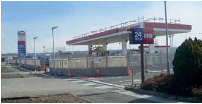
Site under construction
