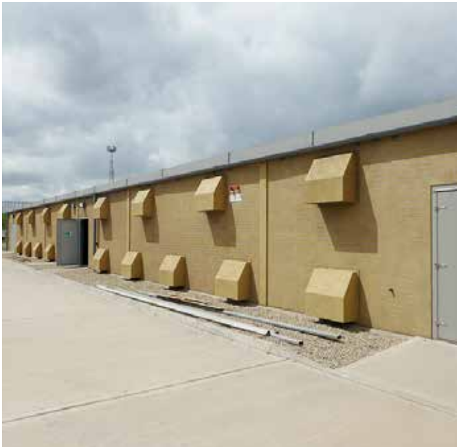
UK gas valve plant
