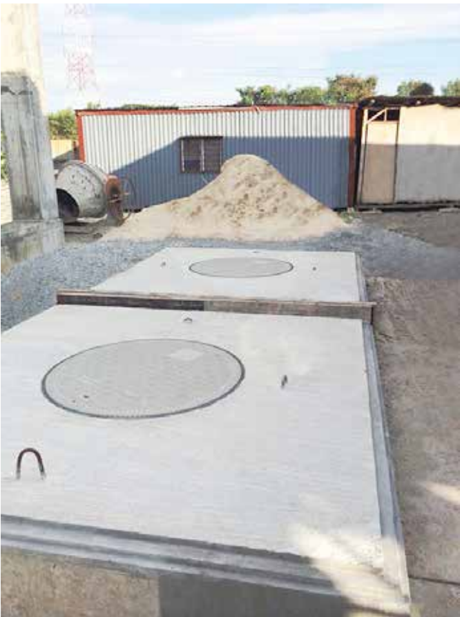
Plinths ready for installation
