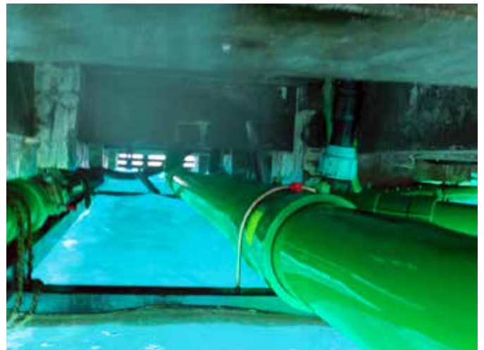
KPS piping is impervious to corrosion from saltwater
