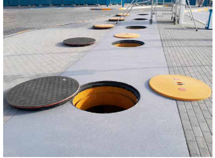
Completed installation with Fibrelite's FL100 (40"/1020mm) watertight lightweight covers
