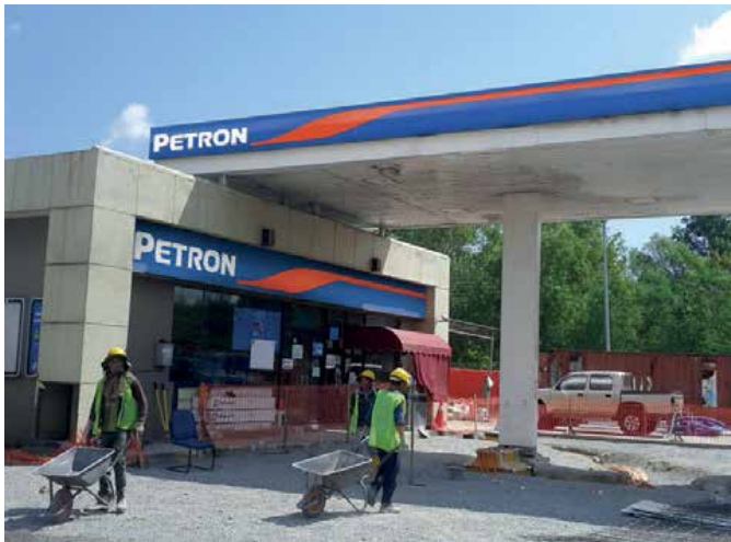
Site under construction
