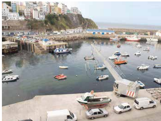
Malpica port now has a safe and reliable piping system thanks to KPS
