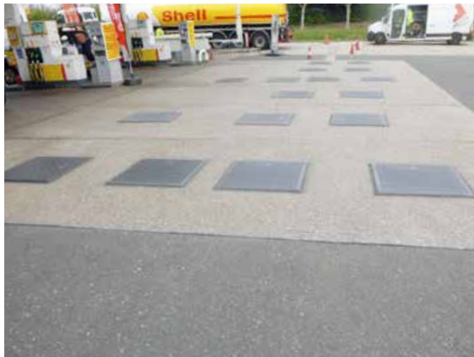
Unusual site configuration with double tank manways
