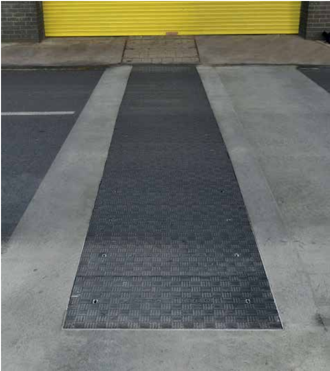
Fibrelite heavy load rated composite trench cover
