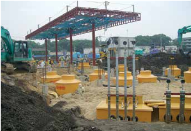
Site under construction
