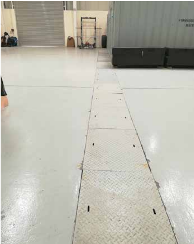
Previously installed steel covers
