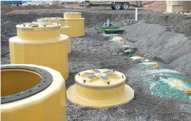
New site in Pennsylvania
