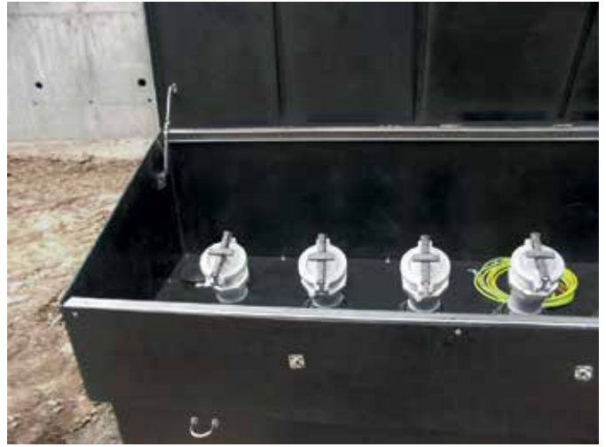
OPW heavy duty corrosion resistant seal caps
