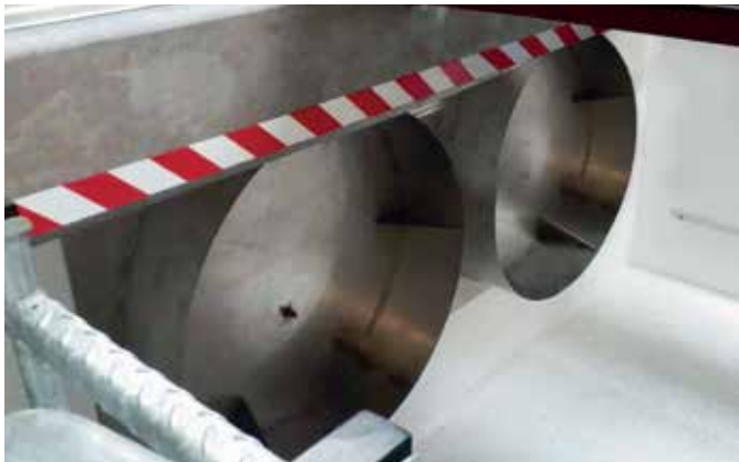
Underground pit to house crane supply lines
