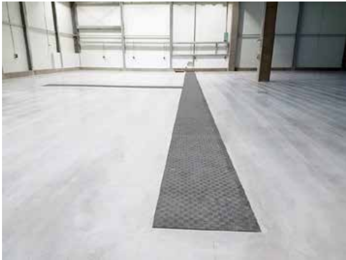
Fibrelite installed D400 covers in a Polish manufacturing facility
