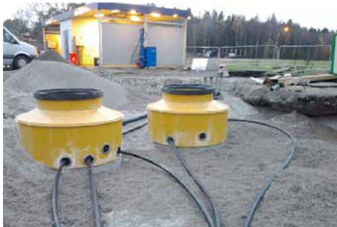
Newly designed 1.7m (S17) diameter tank sumps being installed in Norway
