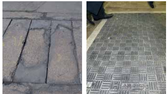
No trips, slips or falls. Fibrelite's GRP composite covers alongside the old concrete trench panels
