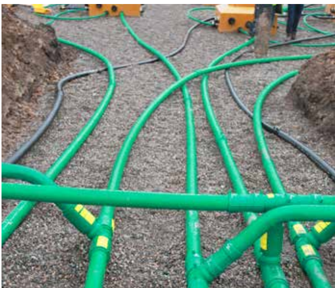
All integrated double wall KPS fittings weld both pipe walls simultaneously
