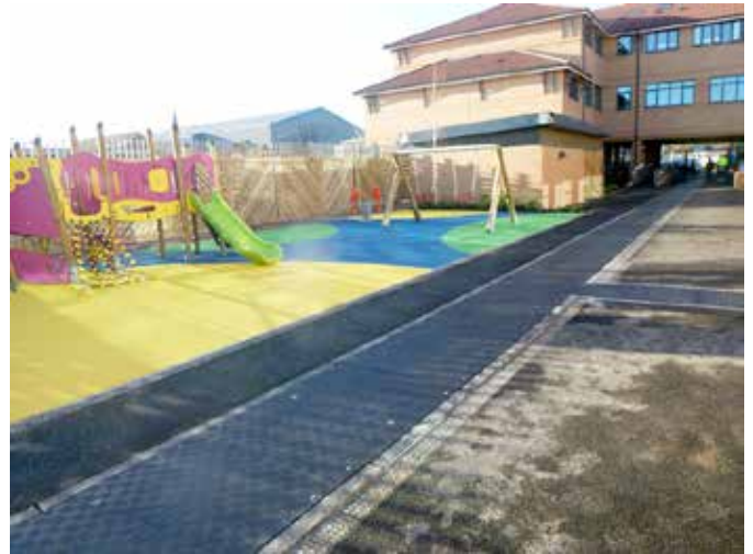
Installing Fibrelite covers helped the site gain the necessary H&S certification
