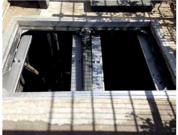
Removable centre beam supports covers
