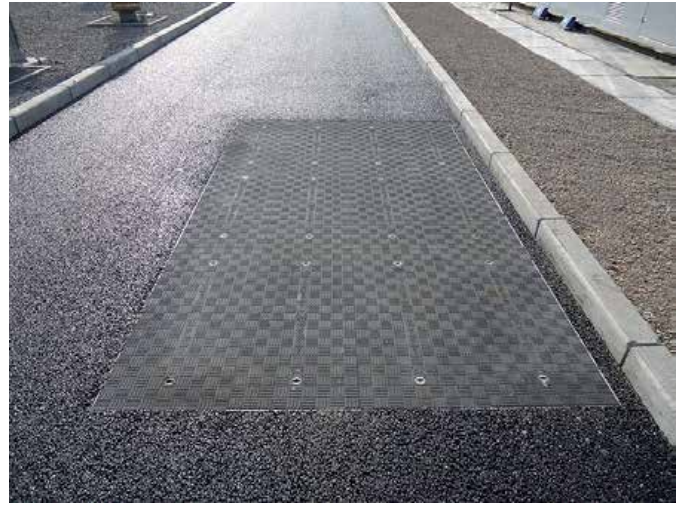
D400 covers installed in an access road on the site
