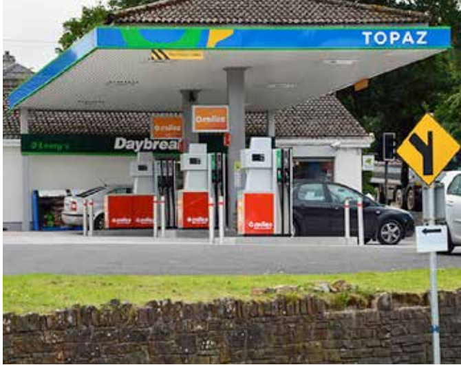
Petro Systems Management has upgraded from steel pipework to KPS
