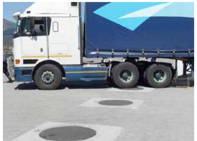
Fibrelite cover installed in truck lane
