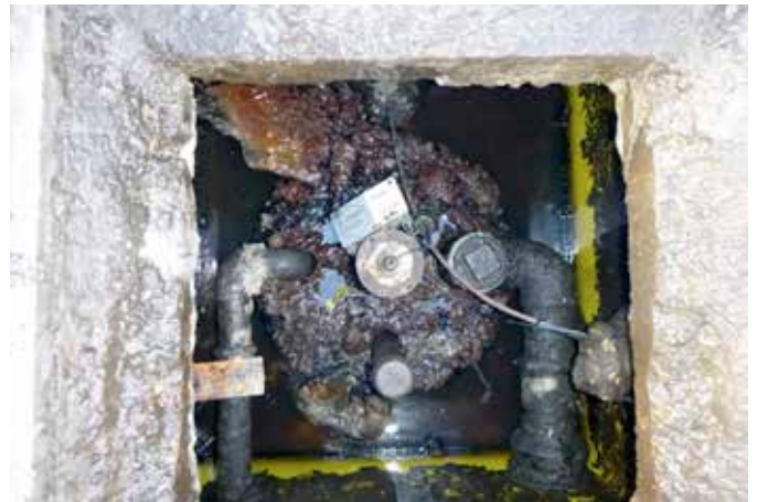
Shell required a retrofit watertight solution
