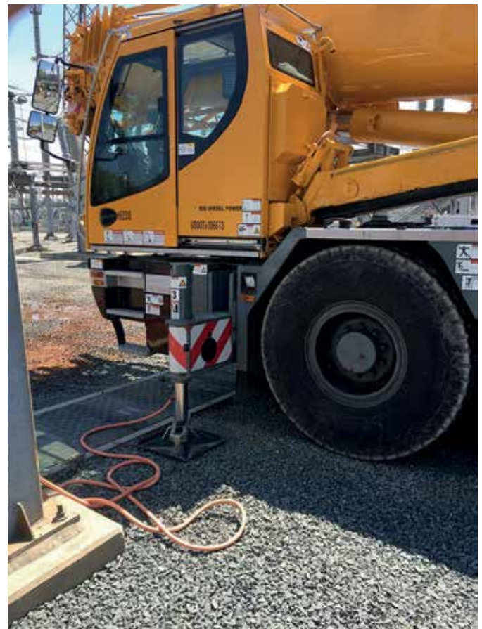
HS-20 load rated trench covers are strong enough to handle an 18 tonne load
