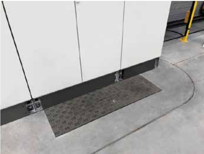
The Fibrelite covers that were installed could withstand loads up to 12.5 tonnes
