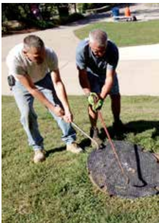
Heavy cast iron covers pose a significant threat of back & shoulder injuries along with the risk of trapped extremities
