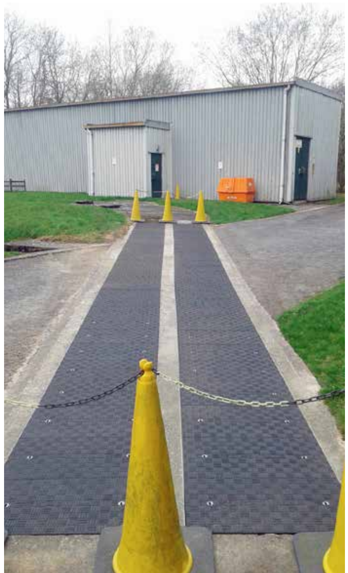
The new D400 load rated covers can be safely removed by two people
