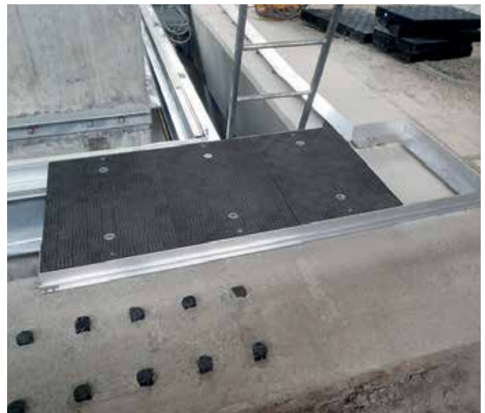
Lightweight tailor made Fibrelite covers set into frame around supporting pier
