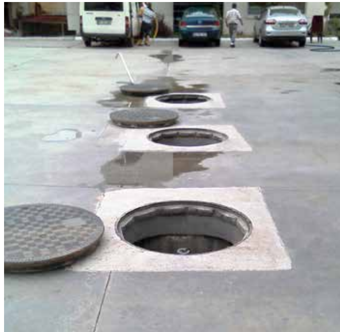
Fibrelite's watertight GRP manhole covers are installed at petrol stations across Istanbul and surrounding areas
