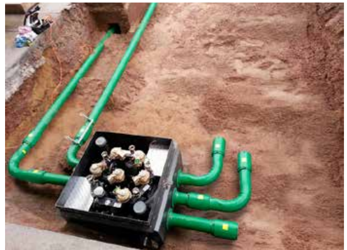
Once the plastic KPS piping was in position, the old steel piping was disconnected and the new KPS piping was connected
