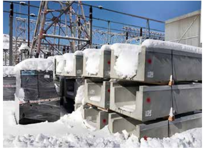
Trenwa's precast trenches ready for installation
