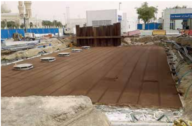
The deep installation required a robust corrosion resistant watertight solution
