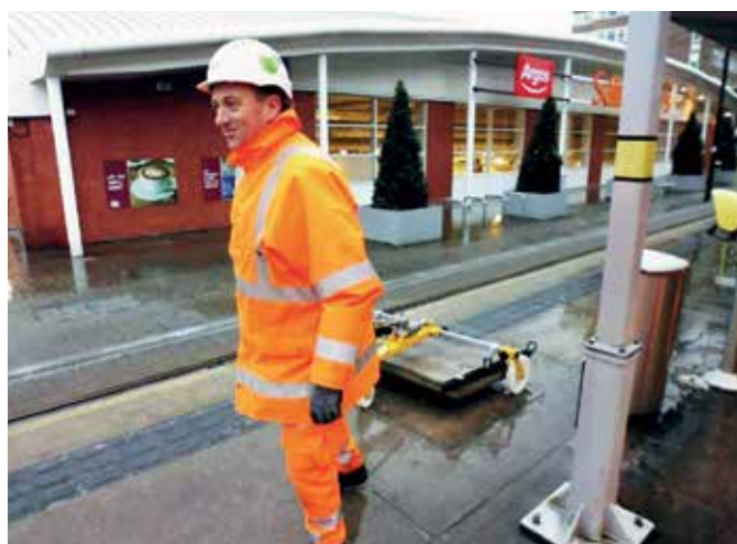
The previously installed heavy concrete covers
