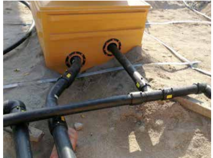
KPS pipework and Fibrelite tank sumps ensure a complete sealed system
