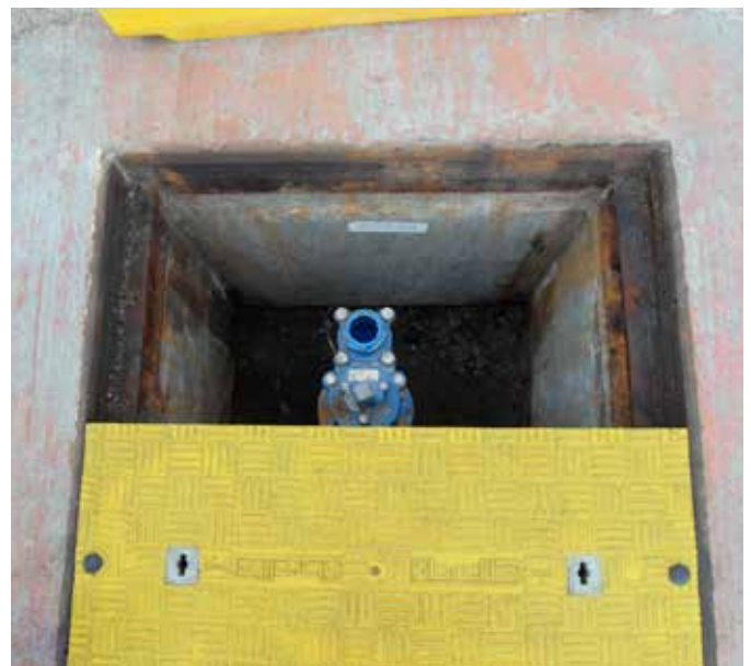
Previously both of the extremely heavy steel covers had to be removed to expose the isolation valve for the drinking water supply. Now only one Fibrelite trench cover needs to be removed
