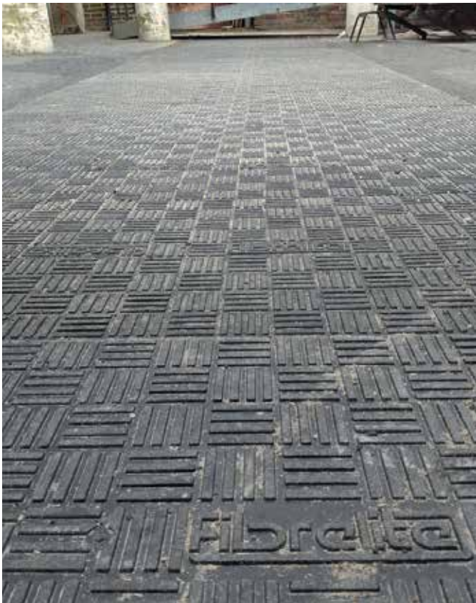
No slips or trips... The Fibrelite tread pattern which offer's anti-slip qualities equivalent to a high grade road
