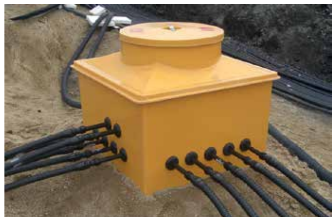
Fibrelite's electrical conduit drawpit being installed
