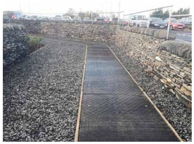
Maintenance free easy to remove Fibrelite covers installed
