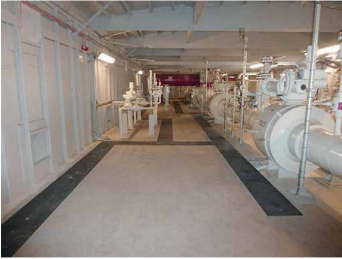
Special notched panels have been fitted around valves and pipework
