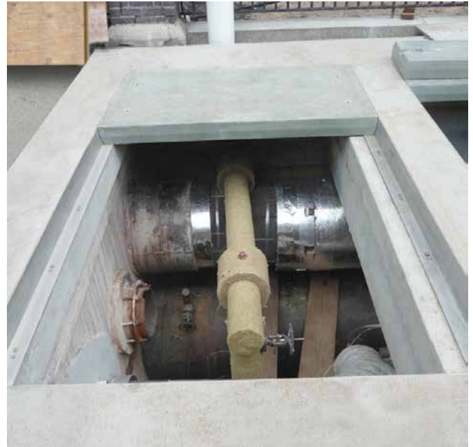
Six Fibrelite FM45 4' 6" (1.6m) wide anti-slip GRP composite trench panels being installed in the sidewalk
