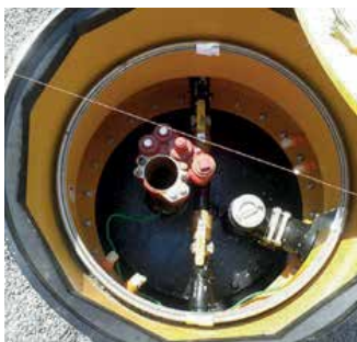
Fibrelite's 1.2m 16 sided turbine sumps being installed
