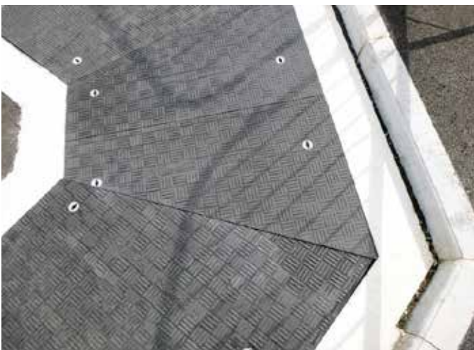
The skid resistant surface of Fibrelite covers removed the potential risk that would have been posed by concrete covers during periods of adverse weather or oil/chemical spillages
