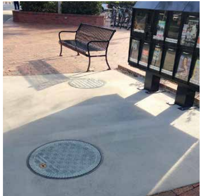
New Fibrelite covers offer a "cool to touch" alternative to cast iron manholes in heavy foot traffic areas.
