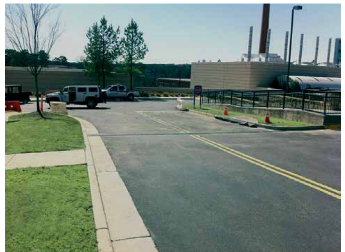
Completed project with Fibrelite's heavy duty covers installed.
