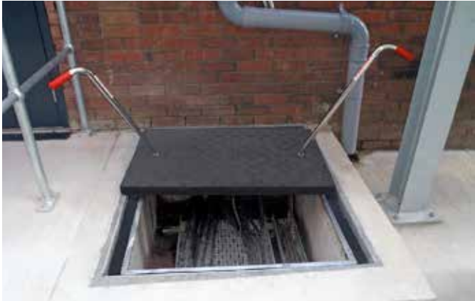
Sealed Fibrelite covers prevent water ingress
