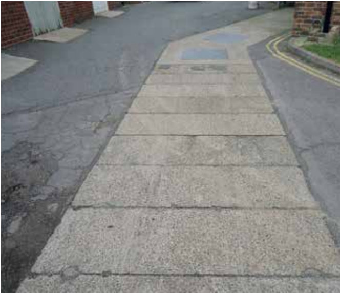
The previously installed run of concrete trench covers
