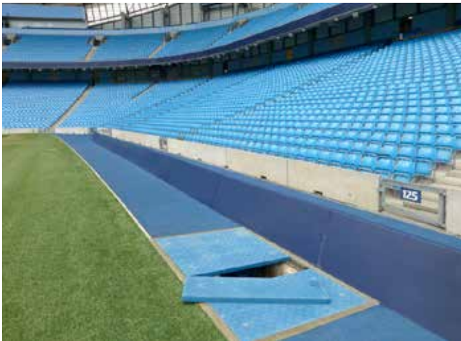
Fibrelite trench covers have an anti-slip surface
