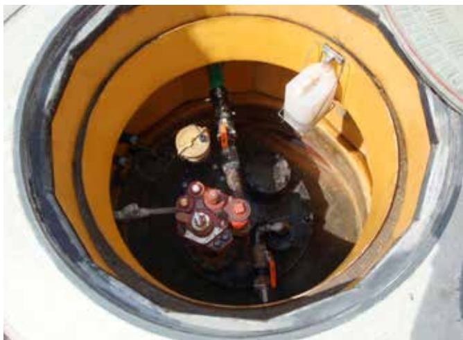
Fiberglass turbine sump with 55" tank collar
