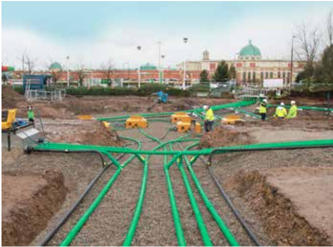
North England site under construction
