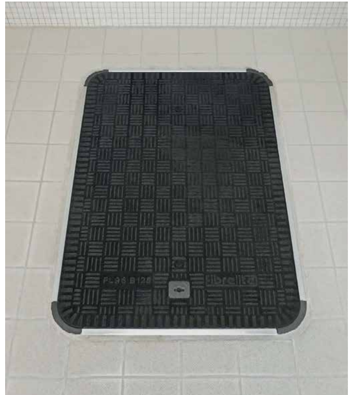
Fibrelite's FL96 watertight manhole cover installed
