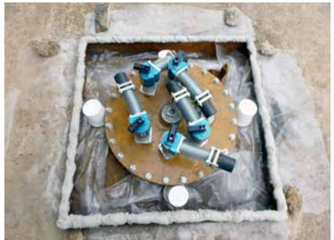
Preparation of surface for putty
