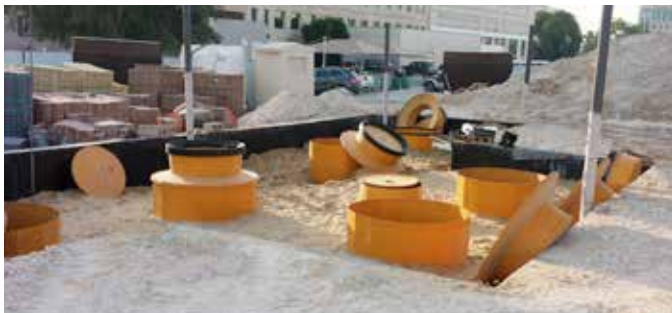
Fibrelite S14-390 tank sumps under installation
