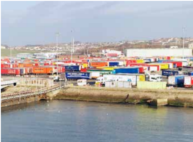
Caption: KPS 125/110mm piping installed at Heysham Port, UK
