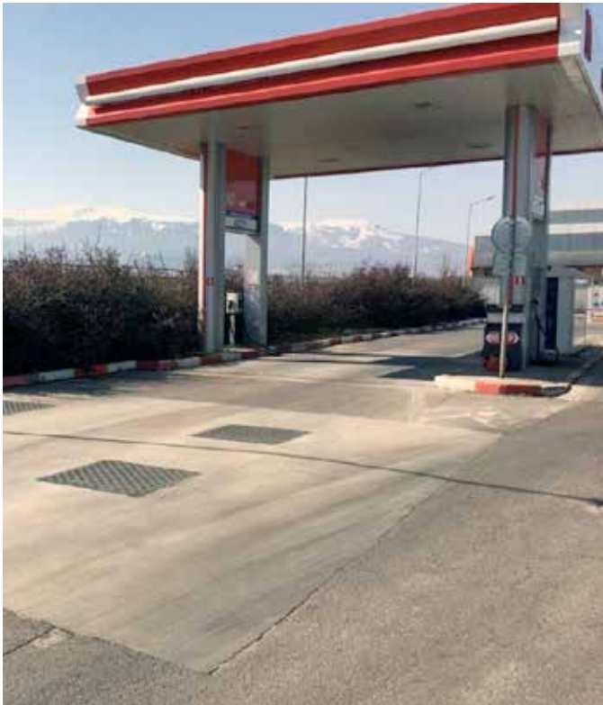
Fibrelite covers installed at a number of LUKOIL sites to replace failing cast iron covers
