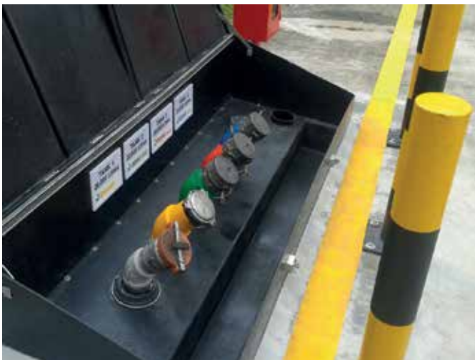
Fibrelite's S22SH-2/AGF above ground remote fill box
