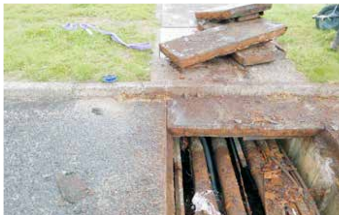
A drill was required for removal and replacement of covers
