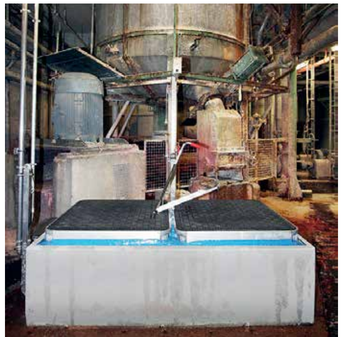
Complete installed Fibrelite covers
