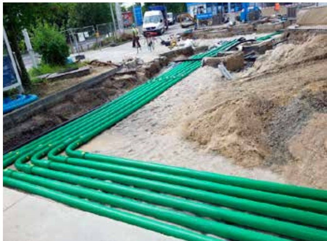
BP-Aral upgrades Leipzig site from steel to KPS plastic double wall piping
