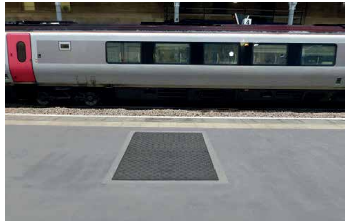
Lightweight Fibrelite covers now installed on platform
