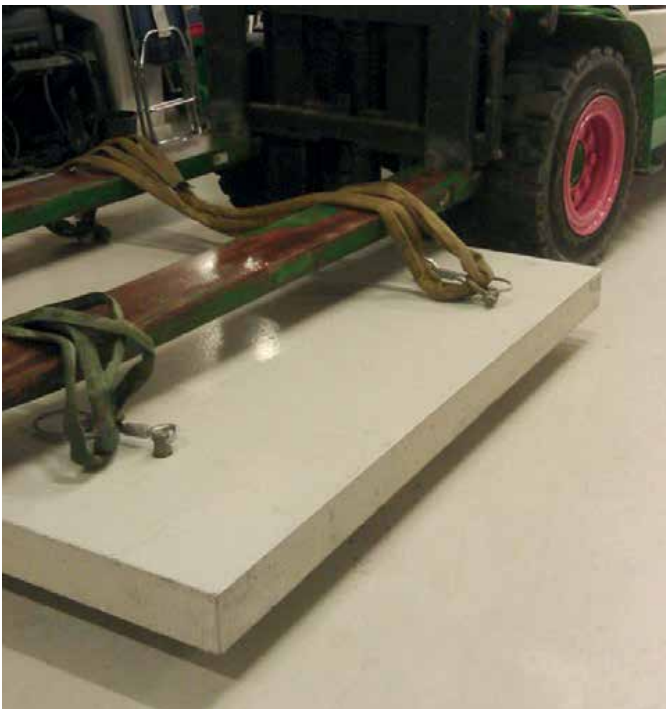
Previously used time-consuming method of removing heavy concrete slab
