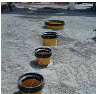
Fibrelite's manual dip and interstitial monitoring sumps being installed
