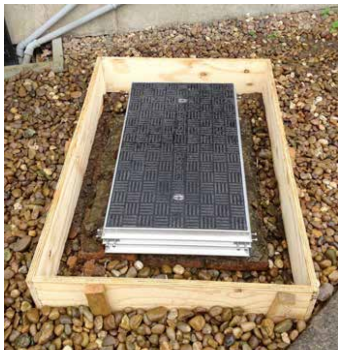
Single FM45 ready for new concrete to be poured
