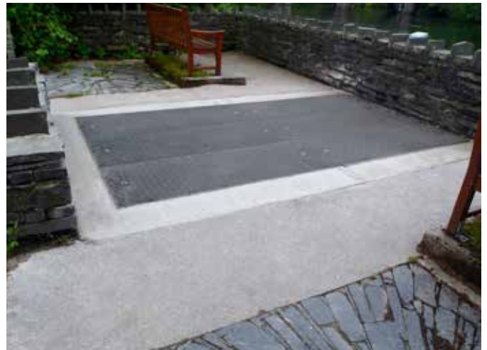
Lightweight Fibrelite trench covers now installed
