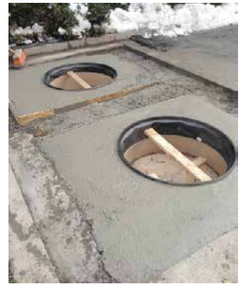
Fibrelite installations are simple – a fiberglass skirt can be used as a preform and to set the frame at grade
