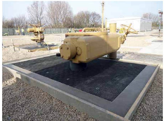
Essential cut outs and profiling for the pipework
