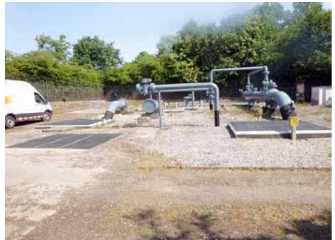
A custom covering solution was required to fit existing apertures and accommodate piping entering trench
