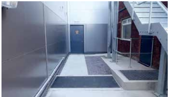
Retrofitted sealed Fibrelite covers installed
