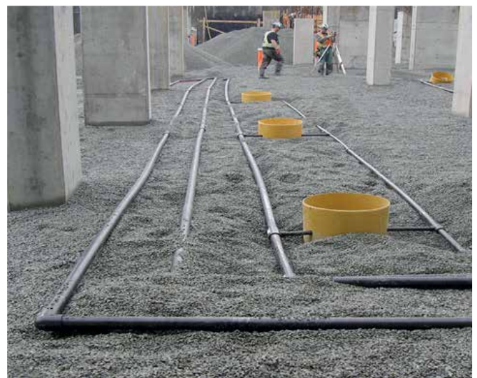
Network of pipes to be buried in the ground
