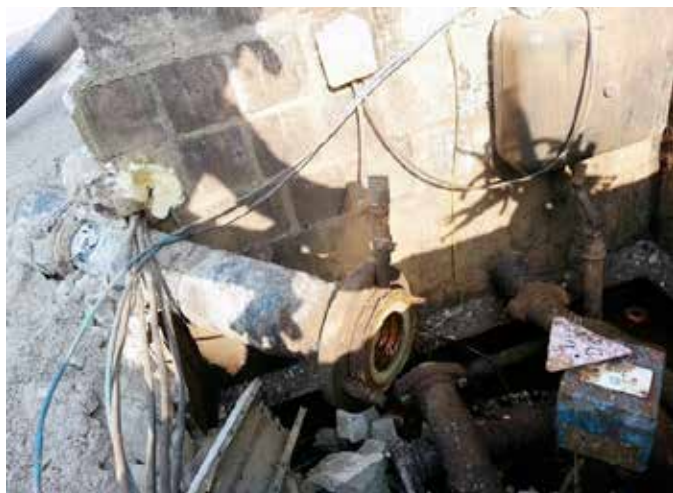
The original piping had been installed over twenty years ago
