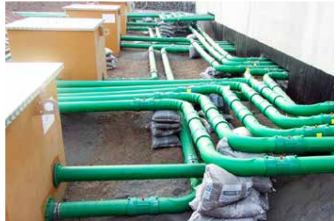
KPS Piping and Fibrelite sumps and chambers were installed
