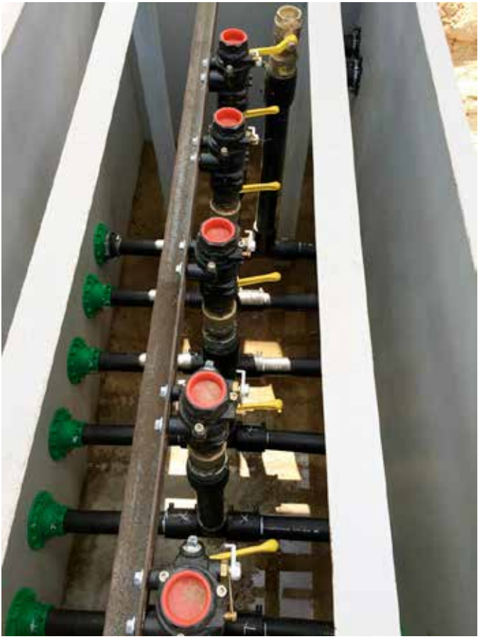
KPS piping combined with OPW shut-off valves creates a reliable fuelling solution
