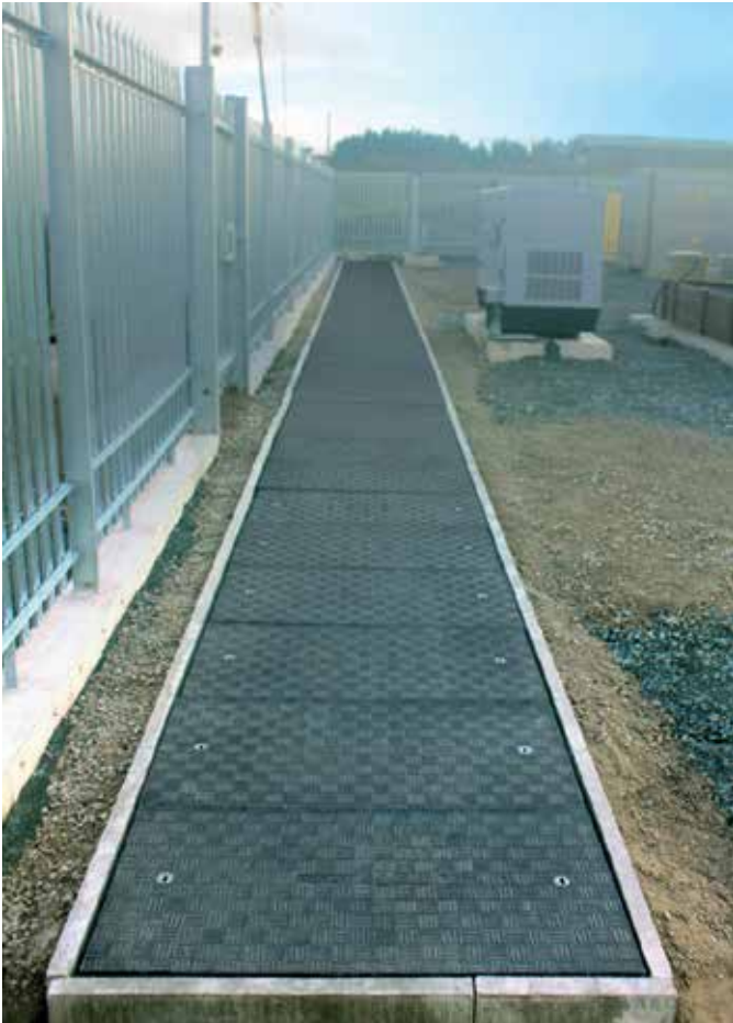
25 metre long precast concrete trench with 1250mm span
