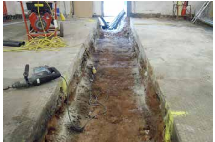
The trenches before Fibrelite install
