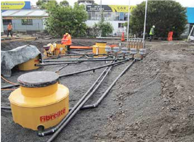
Fibrelite sumps are vacuum testable ensure watertightness
