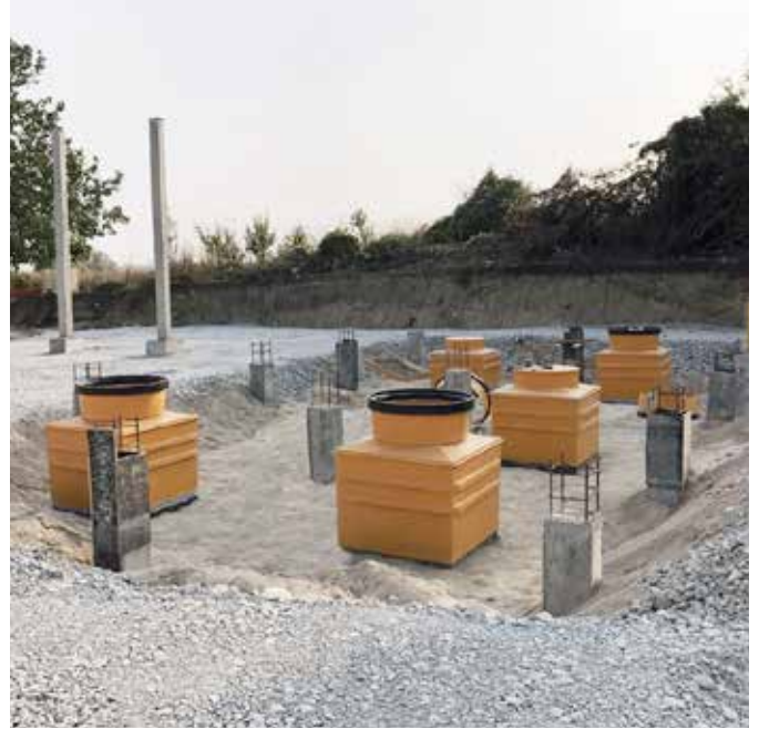
OPW's easy-install Fibrelite below-ground containment can be fit and forgotten for the lifecycle of the site
