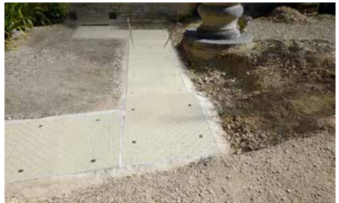
Fibrelite covers prevented the trench from becoming contaminated by debris
