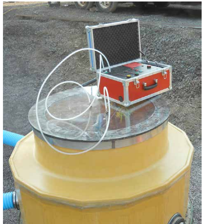
Vacuum testing to ensure a watertight installation
