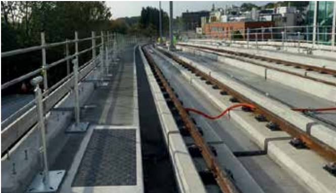
The Fibrelite B125 (12.5 tonne) load rated medium duty trench access covers
