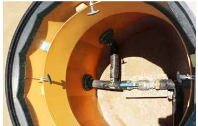
Fibrelite pipe entry sealkits are easy to install, vacuum testable and flexible to allow for ground and pipework movement
