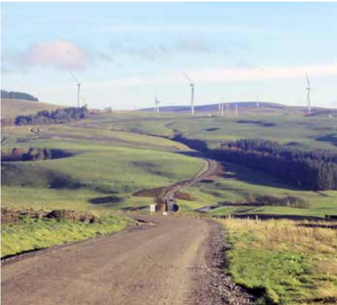
Garreg Lwyd wind farm under construction
