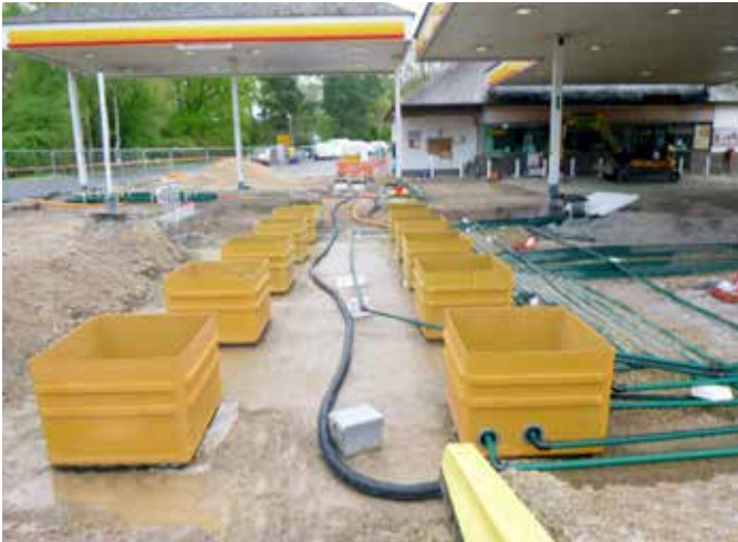
Fibrelite tank sumps bonded to existing tanks using bespoke bonding system
