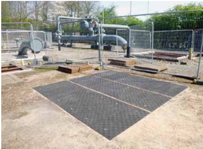
Fibrelite's "fit and forget" retrofit replacement for previously installed eroding concrete covers
