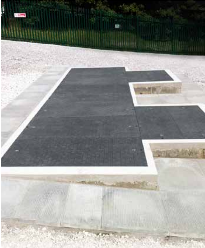
These bespoke trench covers were custom designed to offer easy access to the entire trench
