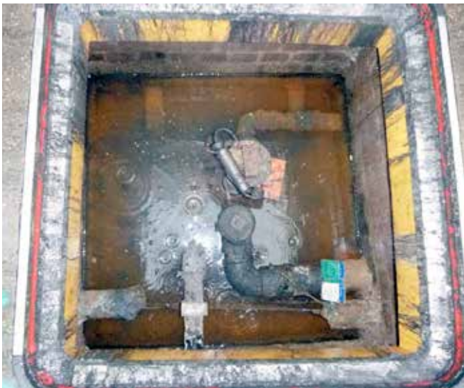
Previously installed brick chambers
