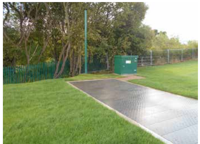
Each Fibrelite cover installed at this site is lockable for added security
