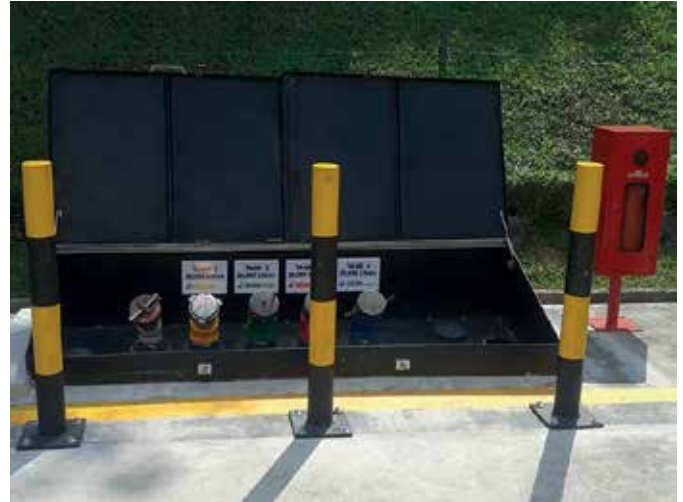
Fibrelite tank sumps being installed
