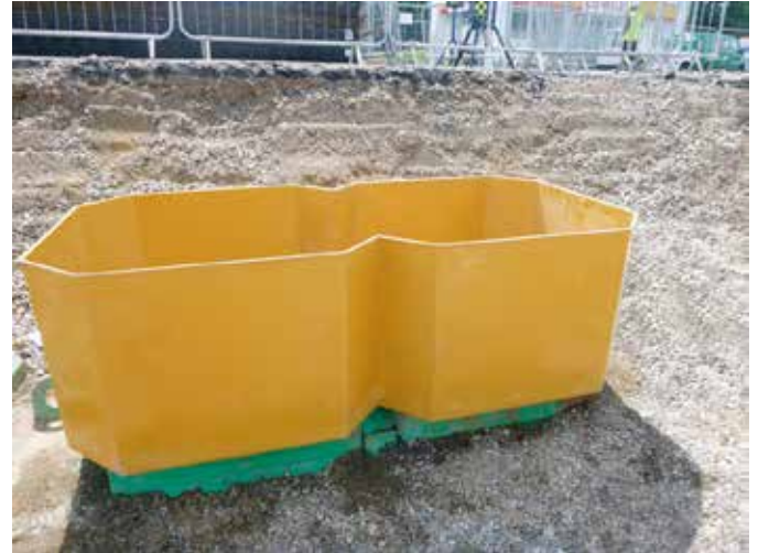
Two Fibrelite S12SQ tank bespoke chambers were fabricated to fit the manway configuration
