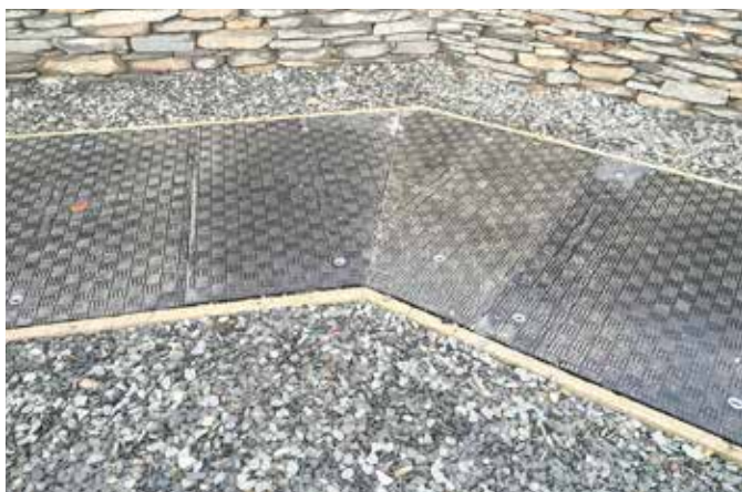
Custom designed and manufactured Fibrelite covers to fit in existing trench
