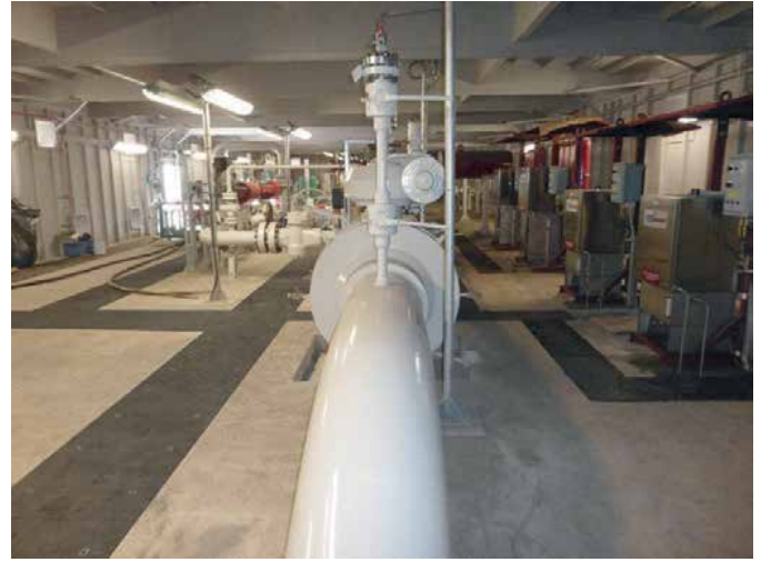
Longer length trenches with no additional support
