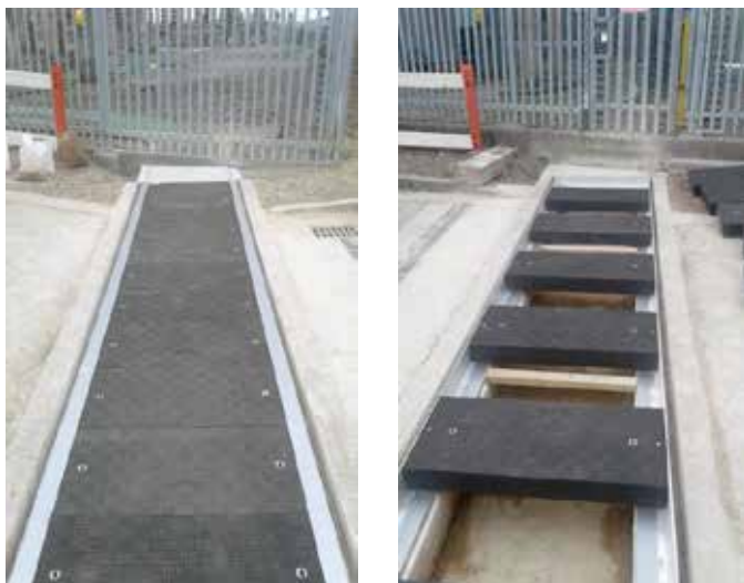
Fibrelite covers and frames were custom made to fit existing apertures, minimising installation time / upheaval to site
