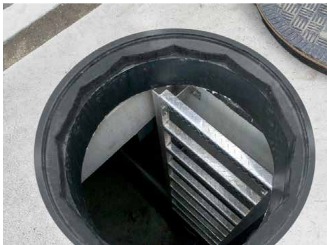
View from over the manhole
