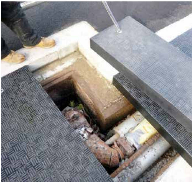
The scale and requirements of this project necessitated a carefully planned bespoke design
