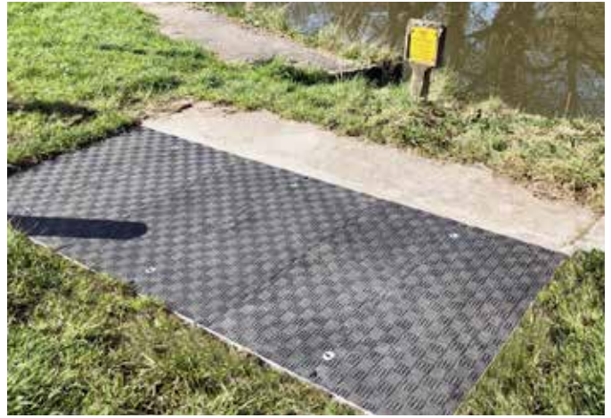
Fibrelite's GRP composite covers have a chemically inert composition and will last for years to come without the need for maintenance
