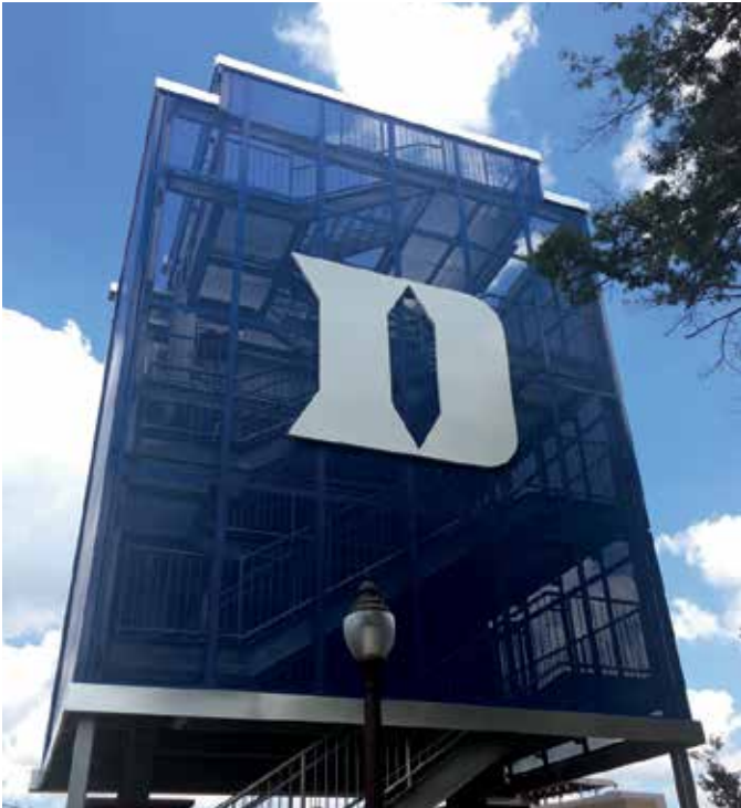
Duke University install Fibrelite trench covers
