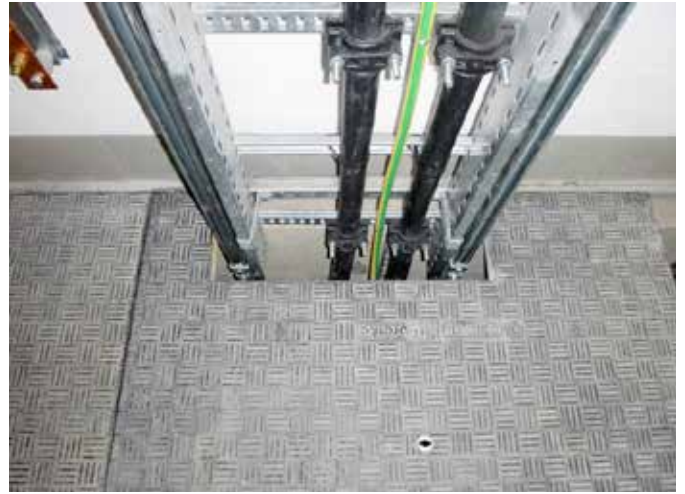
This project had an extremely tight timeline to minimise disruption to the facility
