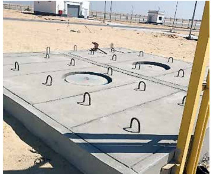
Fibrelite chambers were installed over the diesel fuel tanks
