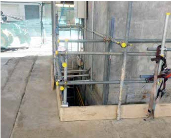
Spherical sliding bearings located in underground pits, allowing for minor movement of the pier
