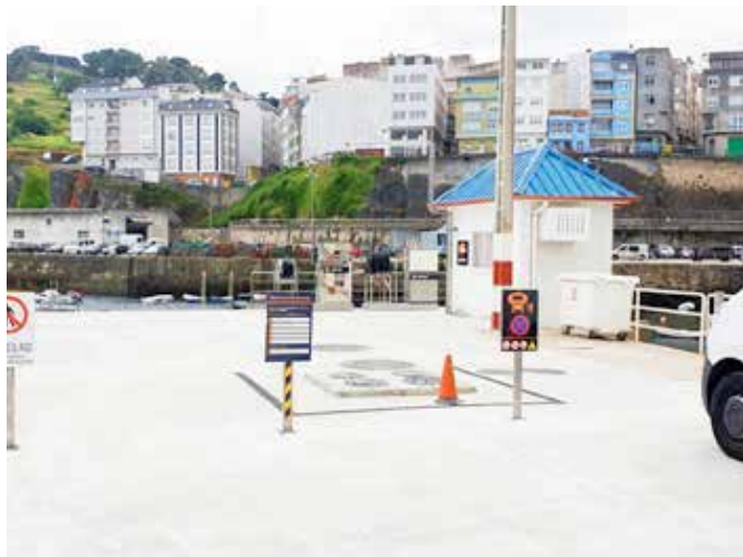
A long-term replacement for corroded metal pipework at Ondarreta, Sada and Malpica ports was needed
