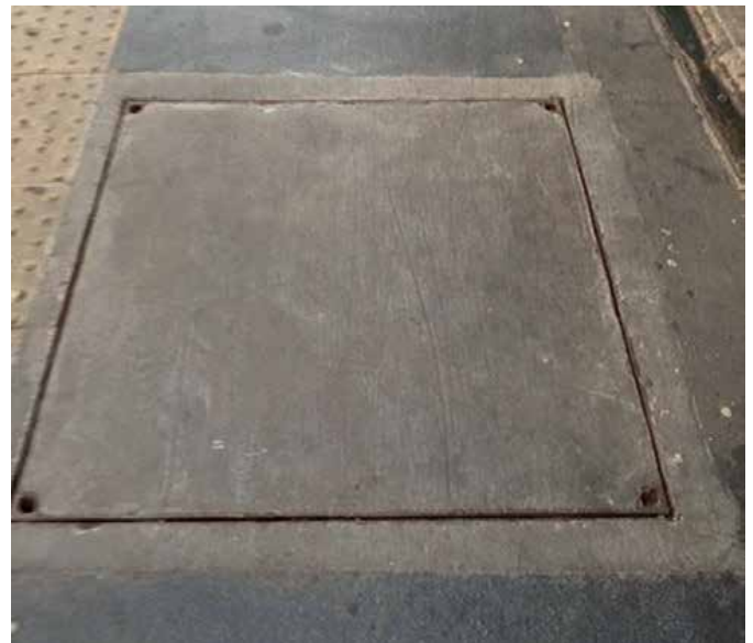
Previously installed, heavy, difficult to lift concrete covers
