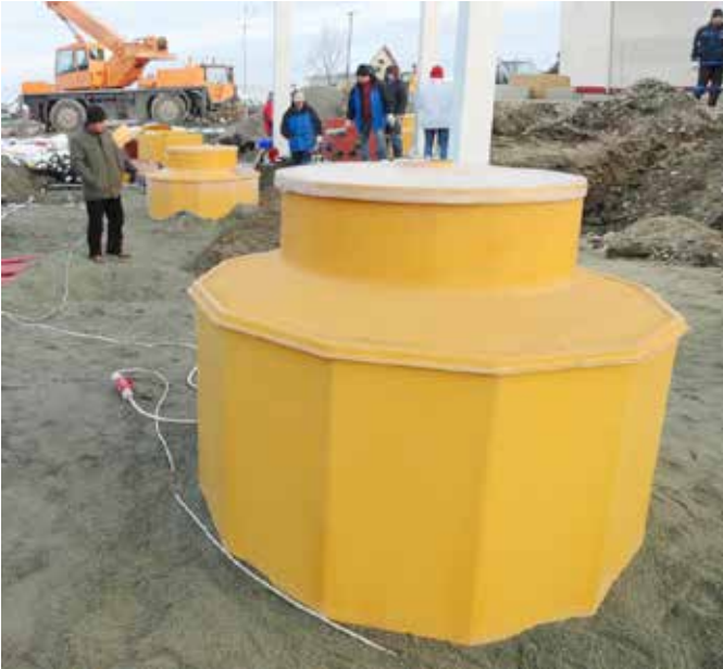
The GRP chambers are fully adjustable to accommodate shallow tank burial depths
