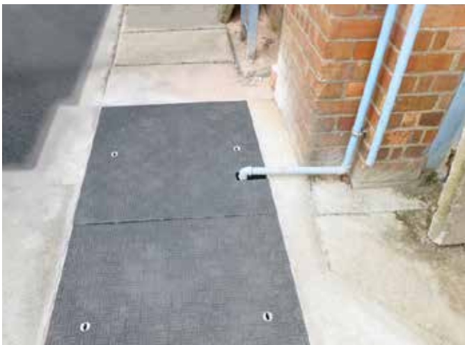
Fibrelite covers provide a lightweight alternative to concrete, alleviating health and safety risks
