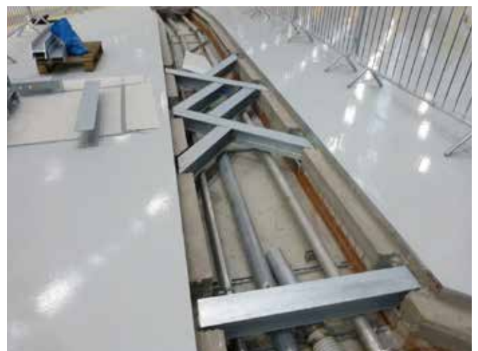
Fibrelite covers needed to be manufactured to work with pre-installed steel supports
