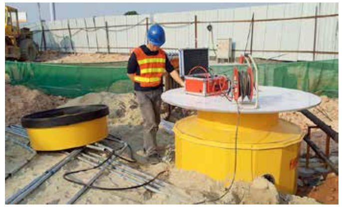
Vacuum tested tank sumps
