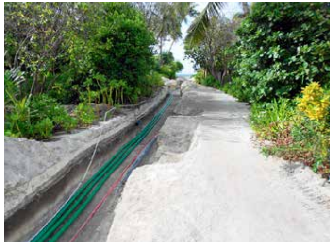
Installed piping from fuelling jetty to storage tanks ready for burial
