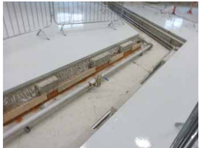
Complex corner trench design
