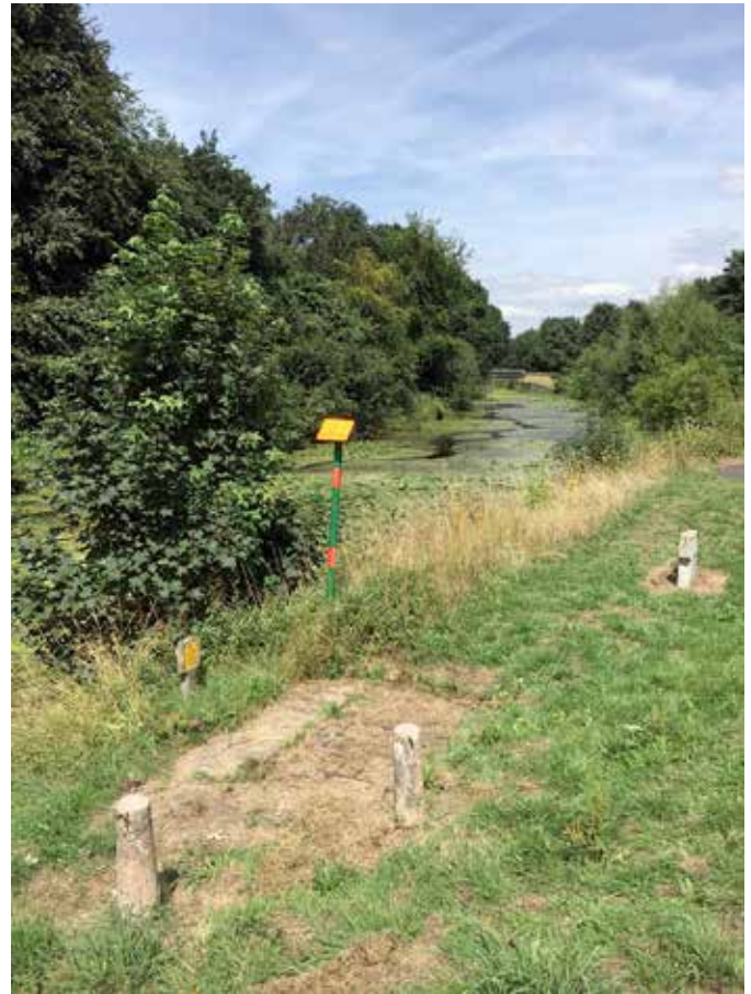
Previously installed concrete infill access covers were causing problems for facilities, especially when it was necessary to gain access to the services beneath
