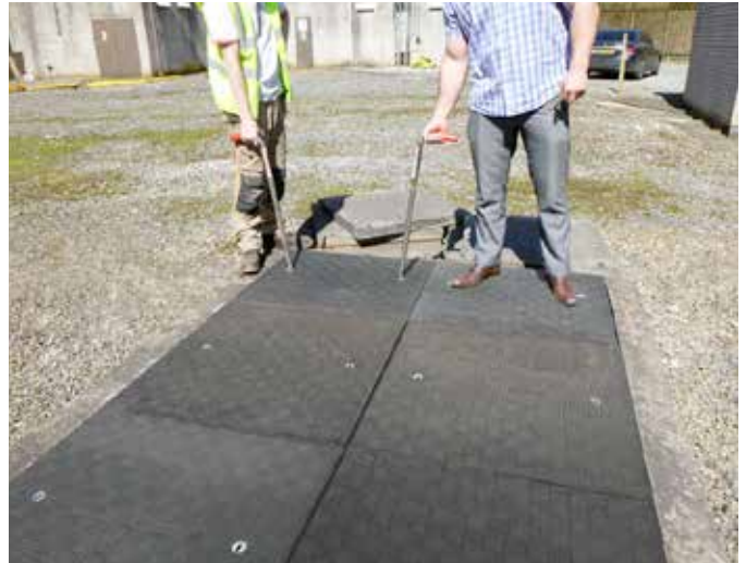
Fibrelite manufactured trench covers which were lightweight and maintenance free
