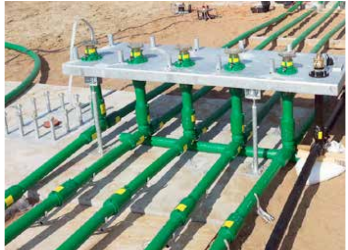
KPS provided an installer friendly solution to meet BP-Aral's strict project deadline
