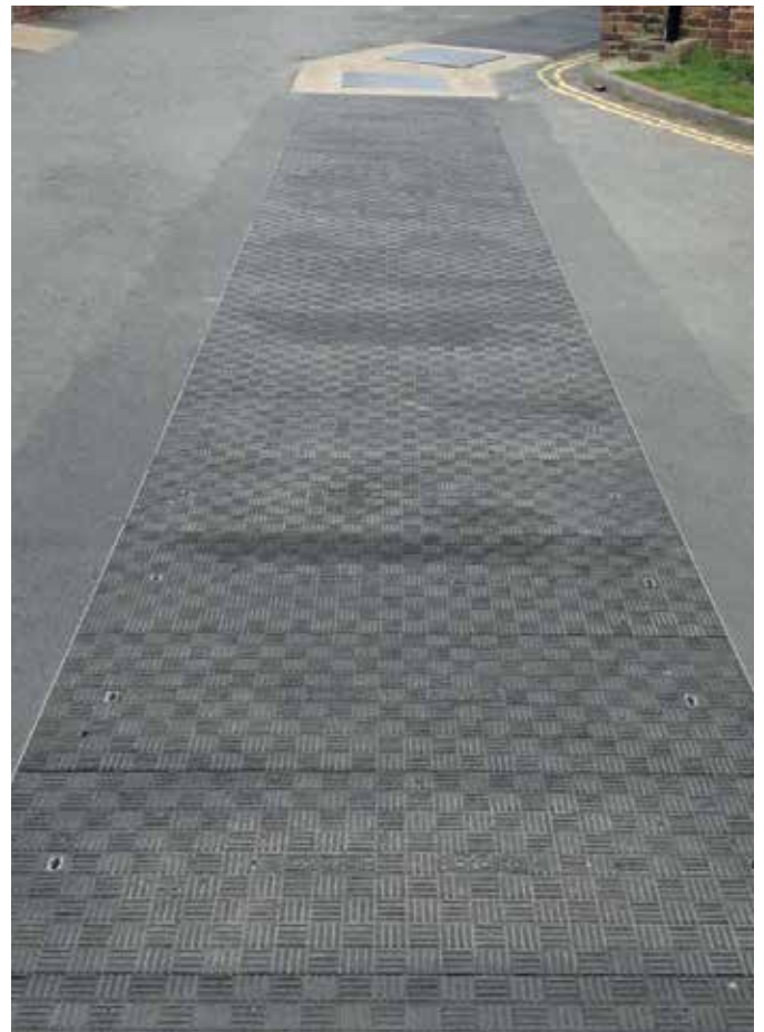
The same stretch following Fibrelite install
