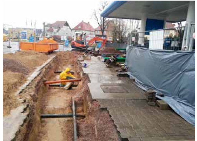
KPS piping was installed one level above the steel piping, preventing interruption of fuel sales
