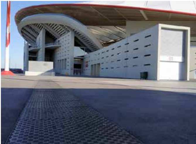
Fibrelite trench covers installed at new Spanish stadium
