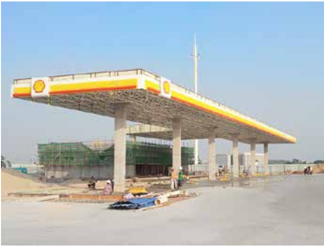
Site under construction
