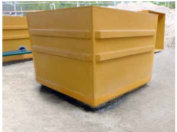
Fibrelite tank sump mounted on old tank upstand
